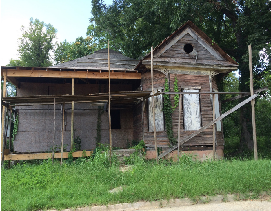
141 E. Cohea St. is another example of one of the few remaining Queen Ann, L plan style houses in the neighborhood. Some one has ensured that this structure remains stable.
