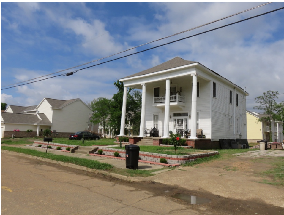
Photo above is of the Greystone Hotel which is individually listed on the National Register. Older photo found on pg.39
