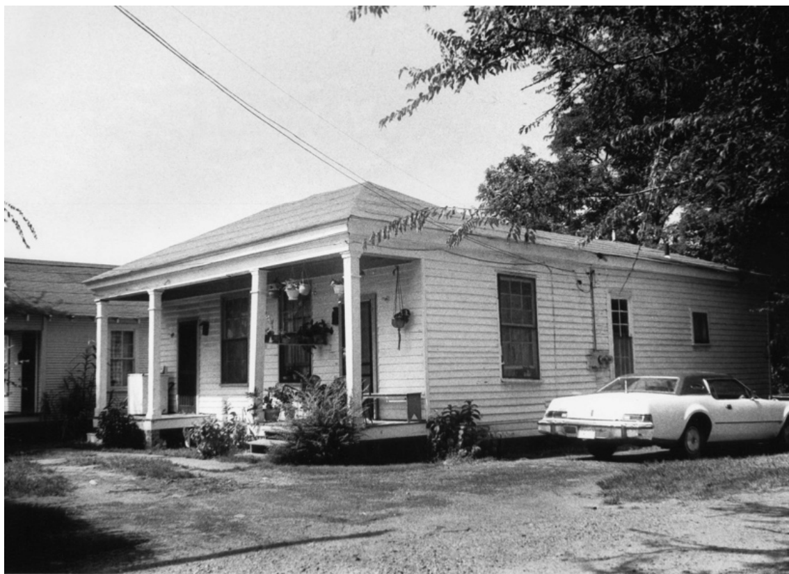
925 Lamar. This house retains Greek Revival style porch posts, shallow hip roof, and 6 over 6 window sash, all features characteristic of vernacular dwellings dating from around 1850.
