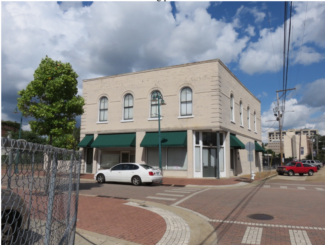
This early commercial building is one of the few in good shape in the District.
