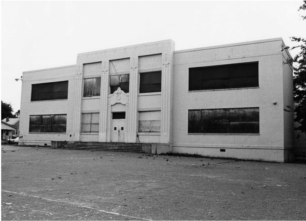
Above photo is an image of the Smith Robertson Museum before its restoration. Photo from National Register Nomination Form, MDAH
