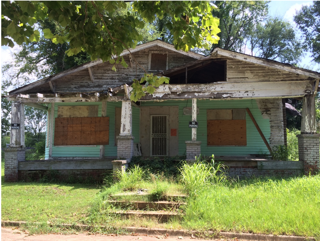
This bungalow at 177 Cohea Street above is in poor shape but appears to be hanging on.
