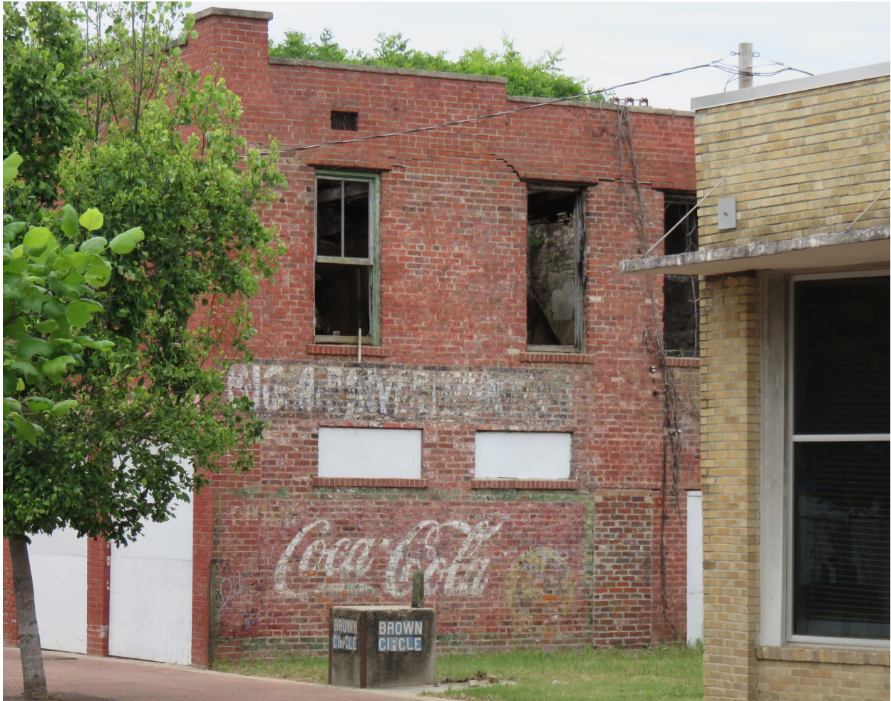
The photo above reveals the poor condition of some commercial buildings on Farish Street in the proposed Entertainment District.
