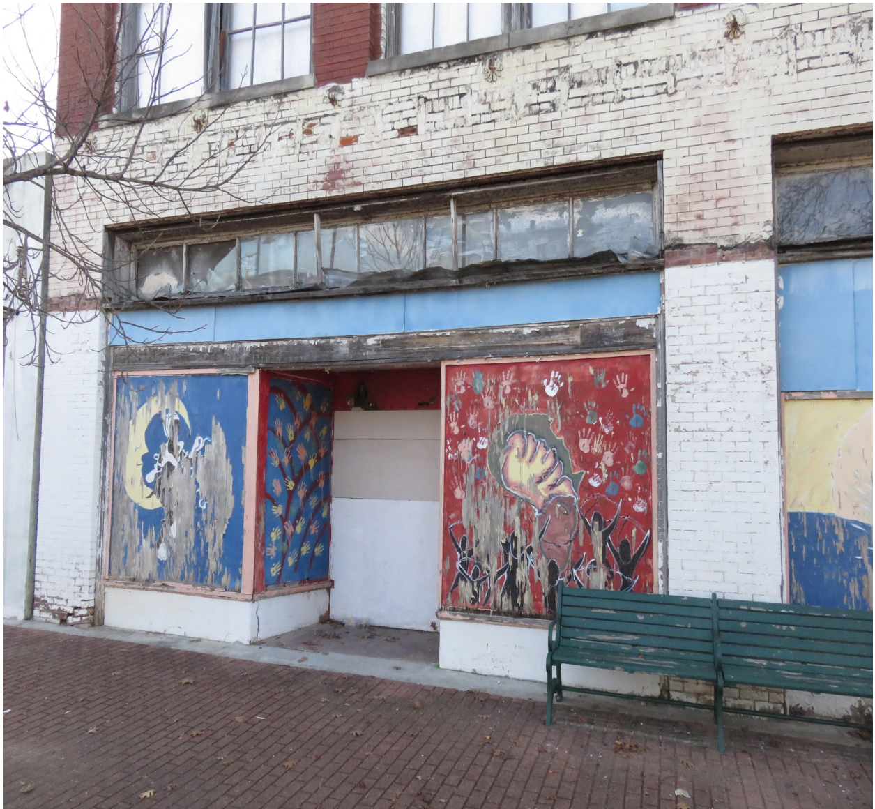
This commercial building has a brick facade, which is peeling away from inner brick wall. Recently it has become unsafe and the city was forced to erect a barrier on the sidewalk below in order to prevent pedestrians from passing by.
