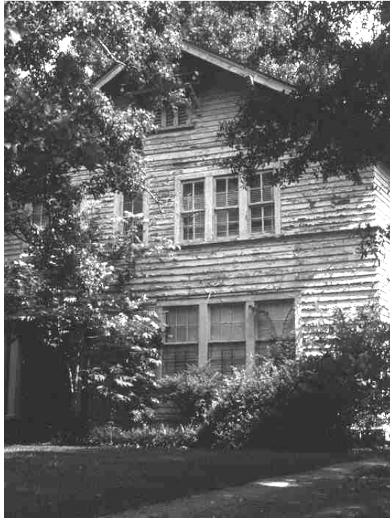
Figure 19. 383 Felder Avenue. Rental Property undergoing demolition-by-neglect
