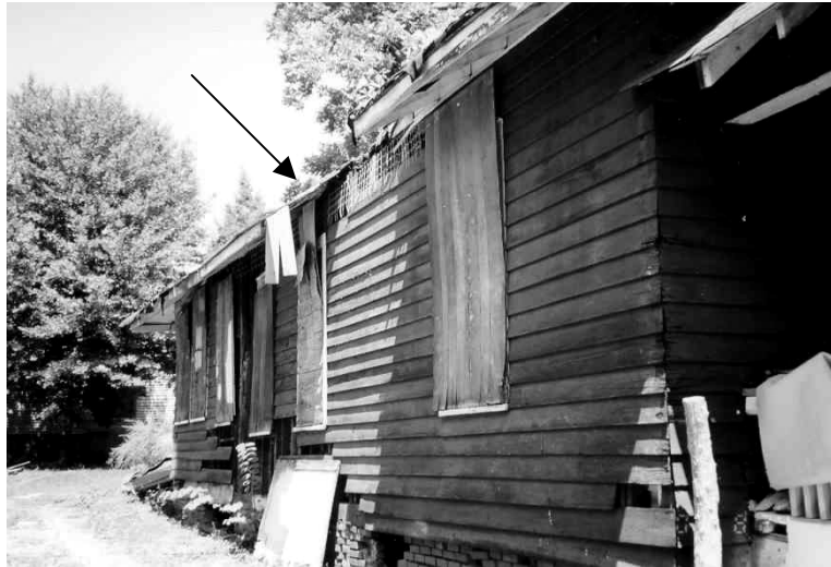
Figure 13. 495 Finley Avenue (August 2002.)
