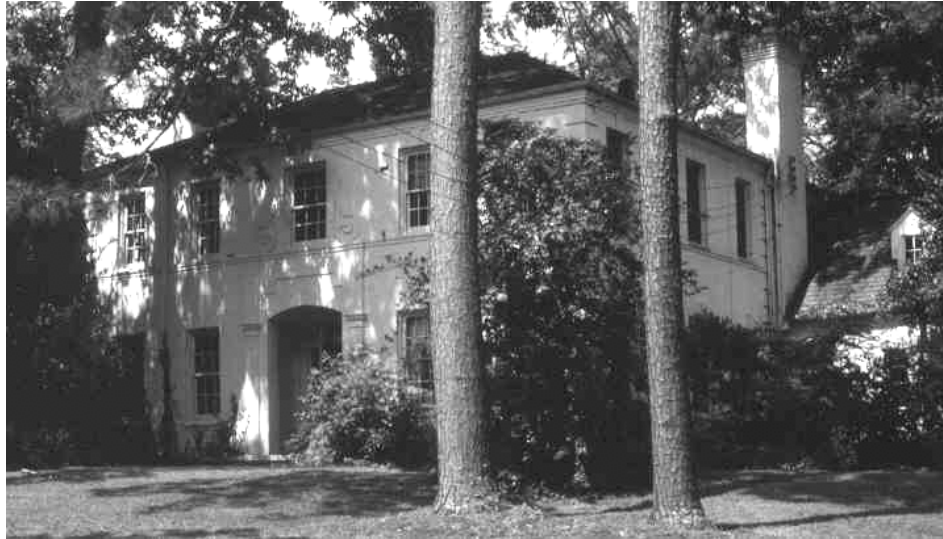
Figure 21. 1826 South Hull - vacant house owned by church at onset of demolition-by-neglect.
