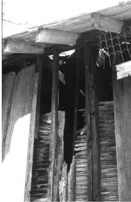
Figure 15. 495 Finley. Open wall one year later due to demolition-by-neglect.
