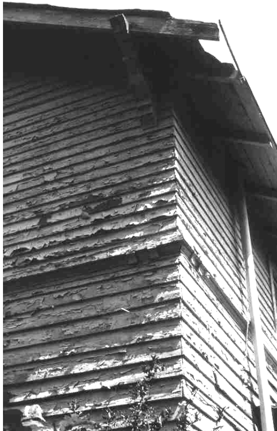
Figure 20. 383 Felder - Peeling paint and eave damage.
