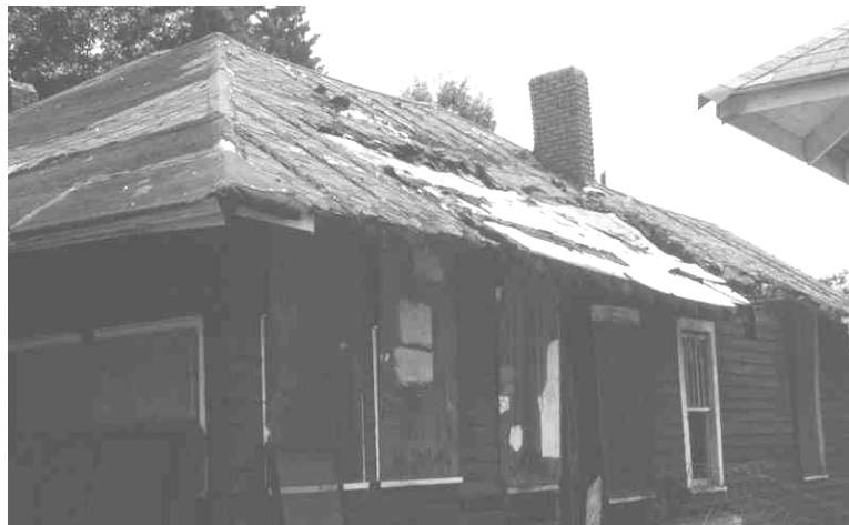
Figure 14. 495 Finley Avenue left unrepaired (July 2003.)
