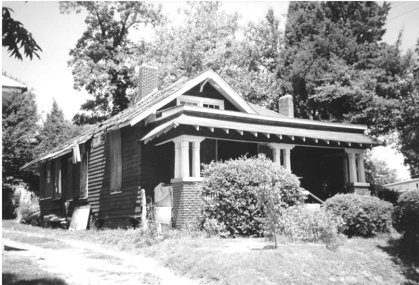
Figure 12. 495 Finley Avenue (August 2002.) Note building is boarded up, structural elements are failing and the building is in disrepair.
