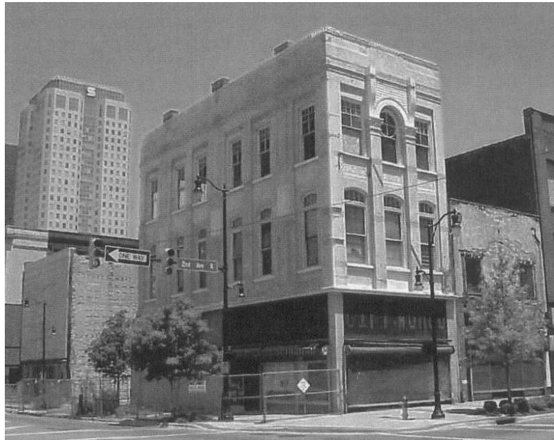
Figure 1. Peerless Saloon (2002) prior to demolition Birmingham, Alabama.
