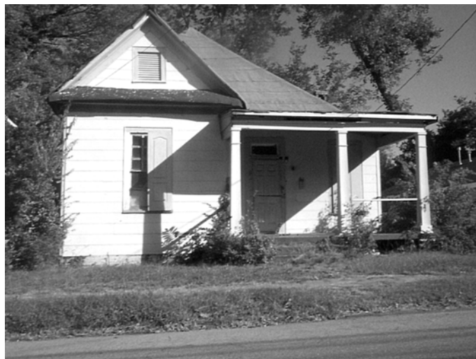
Figure 9. 313 Cramer Street (October 19, 2001)
