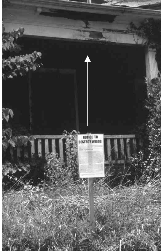
Figure 17. 430 South Highland Court. Arrow points to decay.
