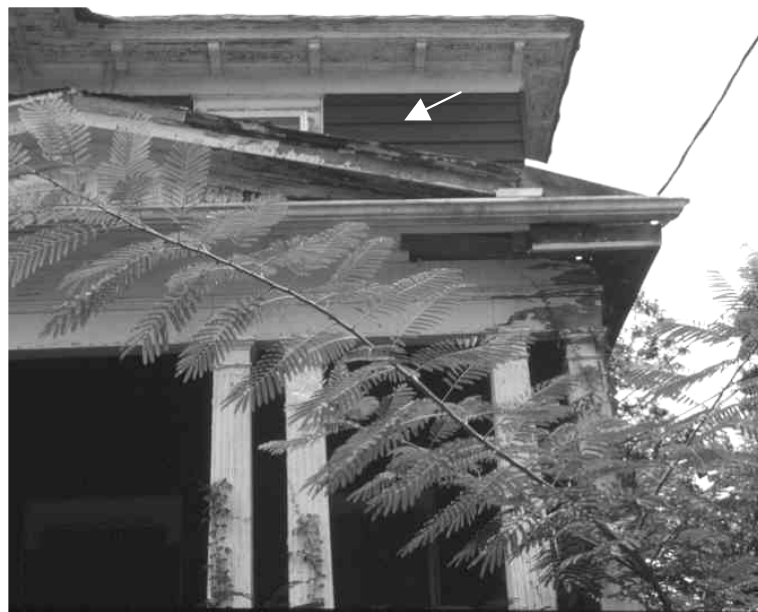
Figure 18. 430 South Highland Court. Porch roof and fascia damage.
