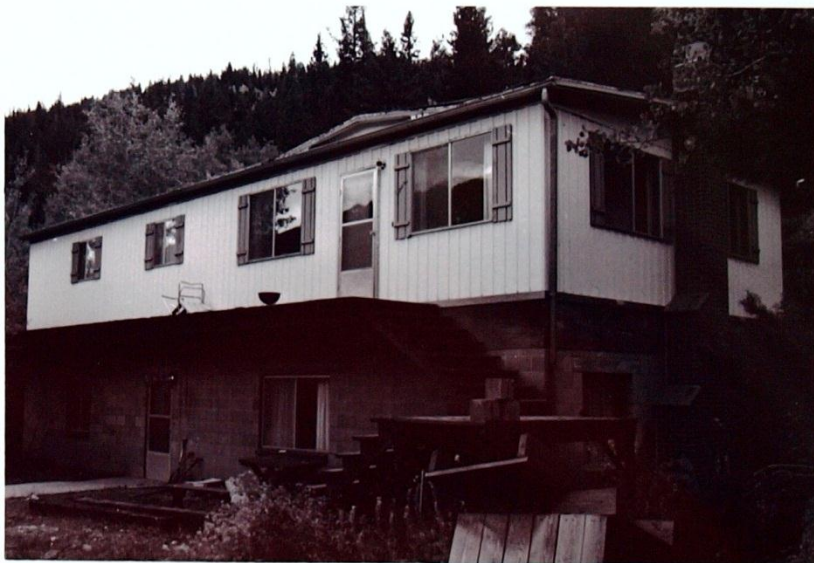
Figure 6.37-demolished residence in Black Hawk Photograph by NPS-RMRO-Denver 1986 Survey Courtesy of the City of Black Hawk
