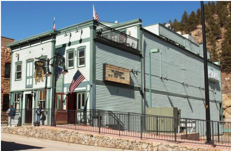
Figure 6.19-Wild Card Casino in Black Hawk Photograph by Deon Wolfenbarger of Three Gables Preservation Courtesy of the City of Black Hawk
