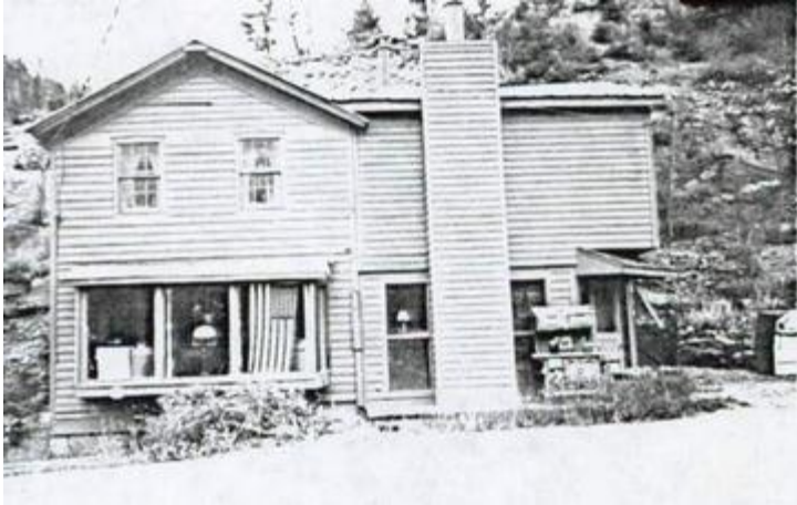
Figure 6.34-Demolished residence Photograph by NPS-RMRO, Denver Courtesy of the City of Black Hawk
