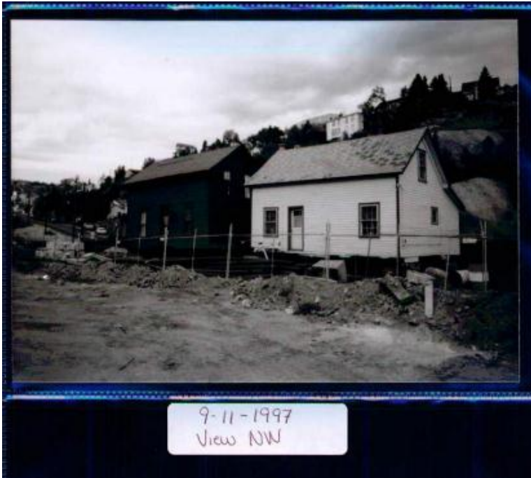
Figure 6.33-420 Gregory Street residence being moved Photograph by Mary Kisling, NPS-RMRO, Denver Courtesy of Central City
