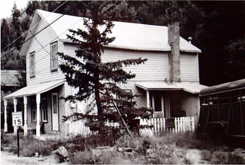
Figure-6.17-Historic Residence at 321 Main Street in Black Hawk in 1986 Photograph by NPS-RMRO-Denver Courtesy of the City of Black Hawk
