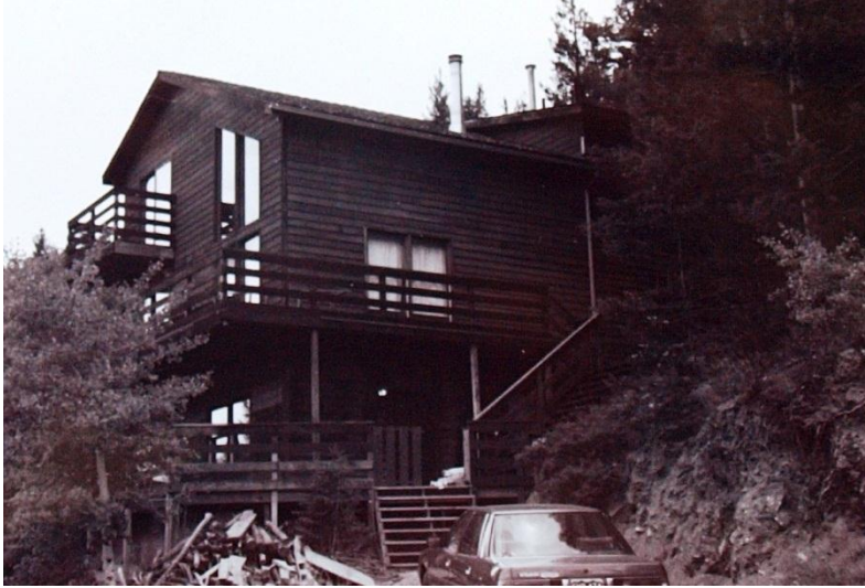
Figure 6.36-demolished residence in Black Hawk Photograph by NPS-RMRO-Denver 1986 Survey Courtesy of the City of Black Hawk
