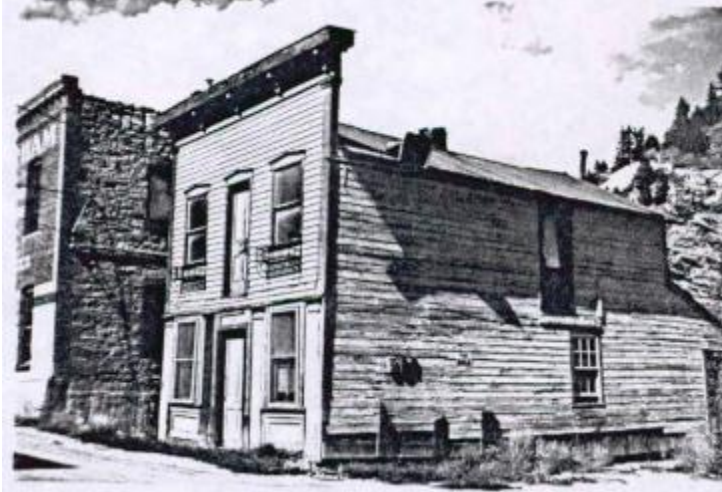
Figure 6.20-120 Main Street in Black Hawk in 1986 Photograph by Rickey Hendricks, NPS-NMRO, September 1986 Courtesy of the City of Black Hawk
