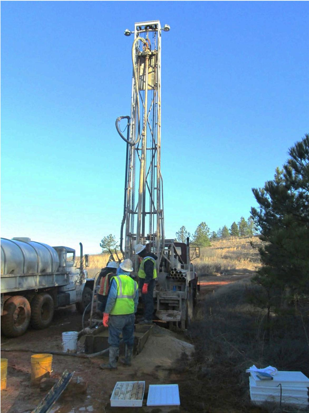
Figure 5. Truck mounted rig and crew drilling through Huber Formation near the intersection of Georgia Highway 17 and Purvis Schoolhouse Road.
