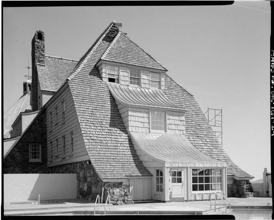
Figure 9.2- “Cat slide” roof on west façade, Timberline Lodge, courtesy of HABS
