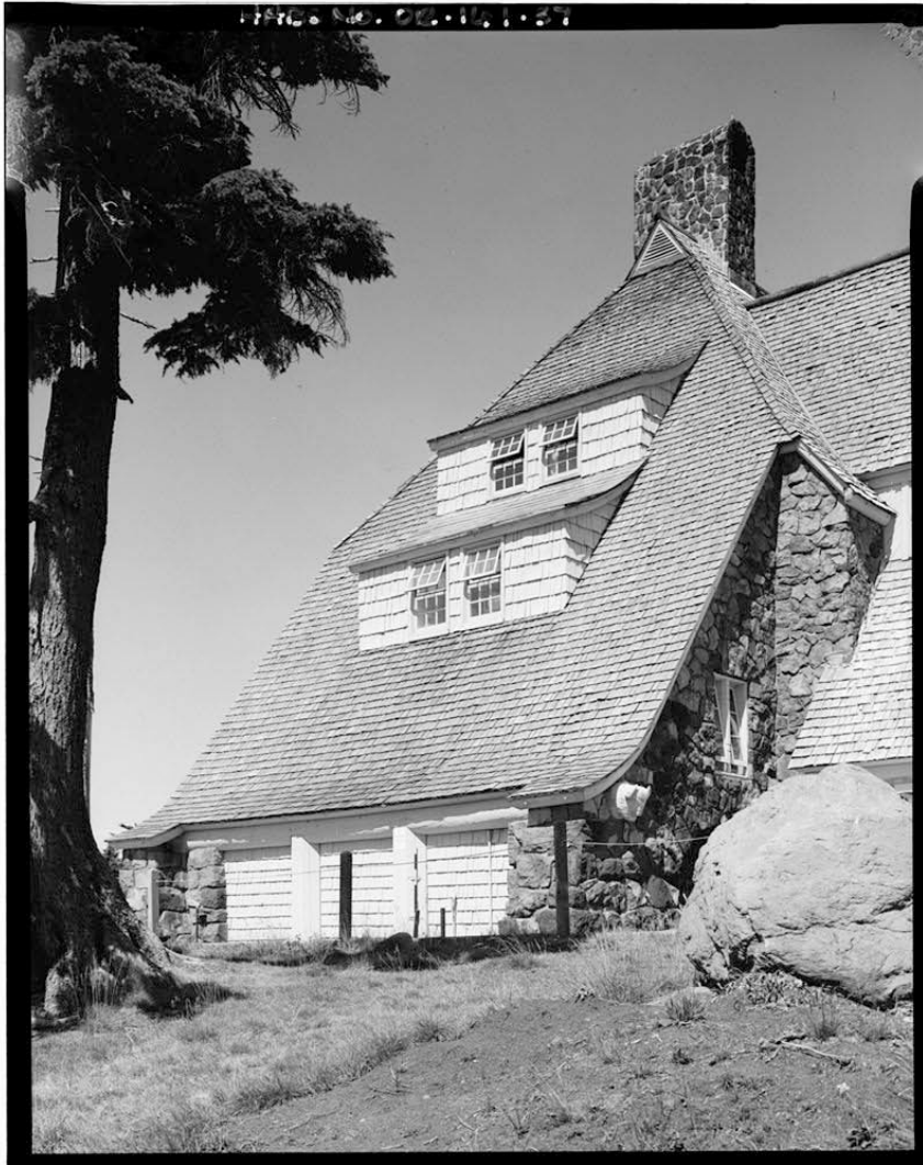
Figure 9.1- “Cat slide” roof on east façade, Timberline Lodge, courtesy of HABS
