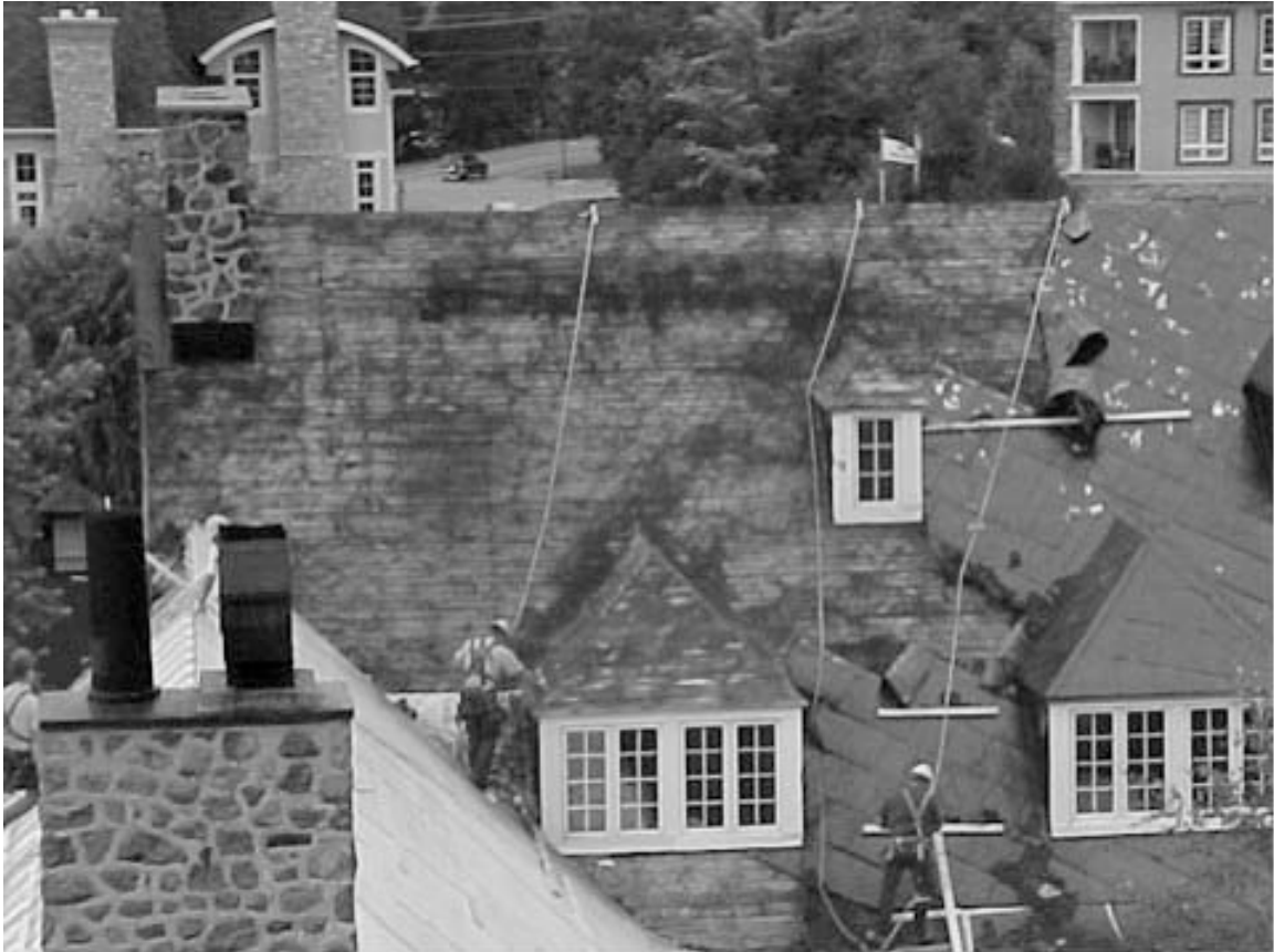
Figure 6.4- Installation of new roof, Tremblant Inn, courtesy of Mont Tremblant
