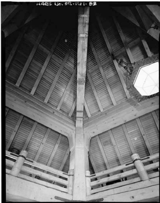
Figure 5.8- False roof detail, courtesy of HABS
