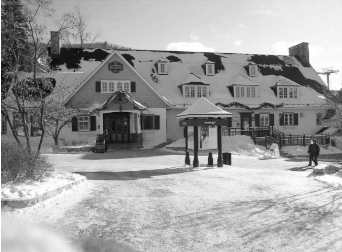
Figure 6.2- Tremblant Inn, courtesy of Mont Tremblant
