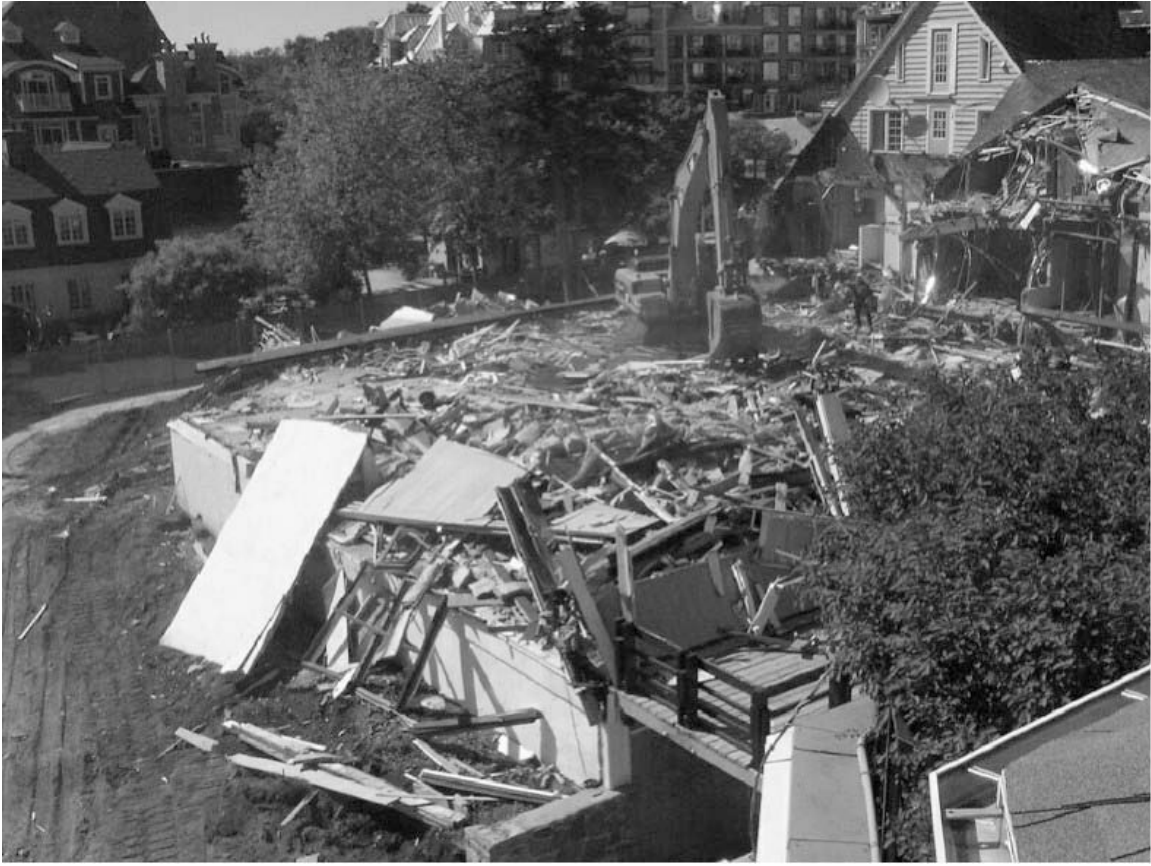
Figure 6.3- Demolition of later additions, Tremblant Inn, courtesy of Mont Tremblant
