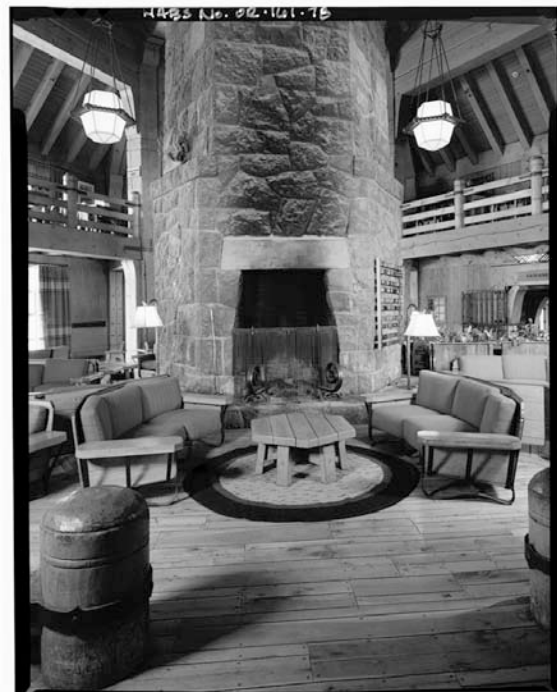
Figure 5.5- Head House Interior, courtesy of HABS
