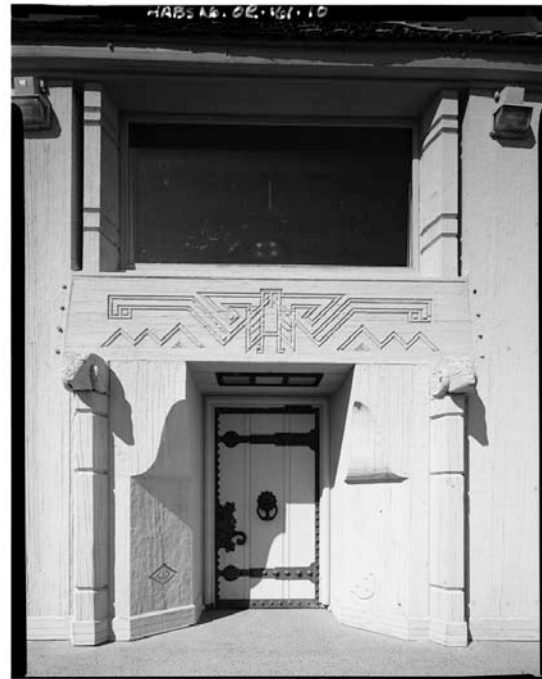
Figure 5.9- Head House entrance and observatory window, courtesy of HABS
