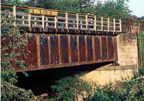
Illustration 4, Mineral Wells-Weatherford Rail-Trail. A rail bridge that has been re-decked for trail use.
