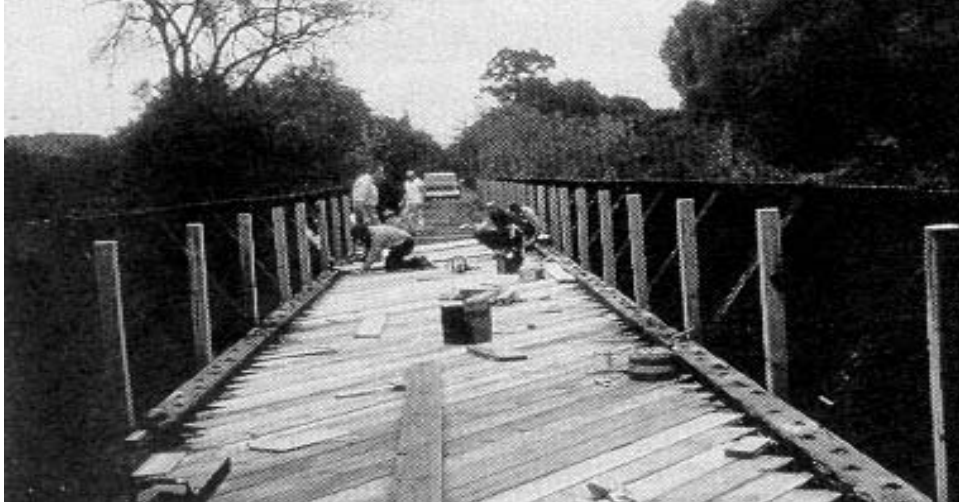
Illustration 14, An example of the conversion of a rail line trestle to a trail bridge.
