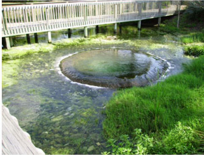
Figure 11.15 – Close-Up View of the Influent Point (Photo by Author).
