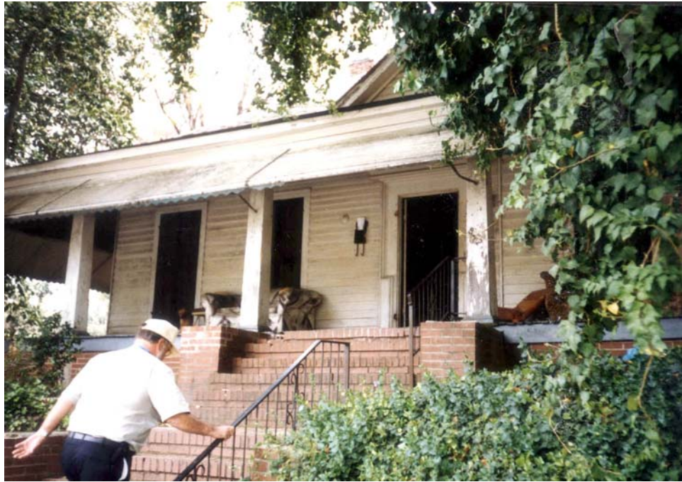
Figure 58: 842 Tatnall Street Before Rehabilitation. (Photograph courtesy of Macon Heritage Foundation)
