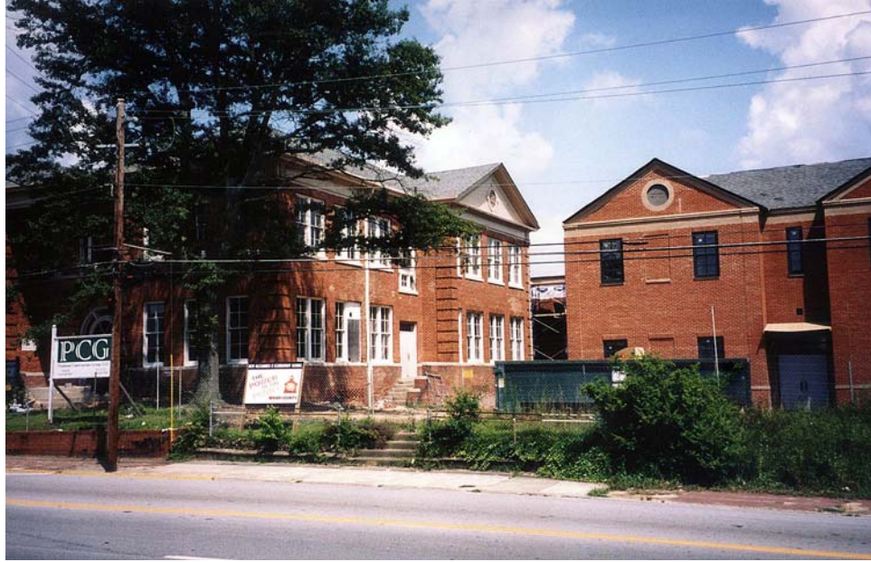
Figure 85: Additions to the Historic Alexander II School Building. (Photograph by author, 2003)
