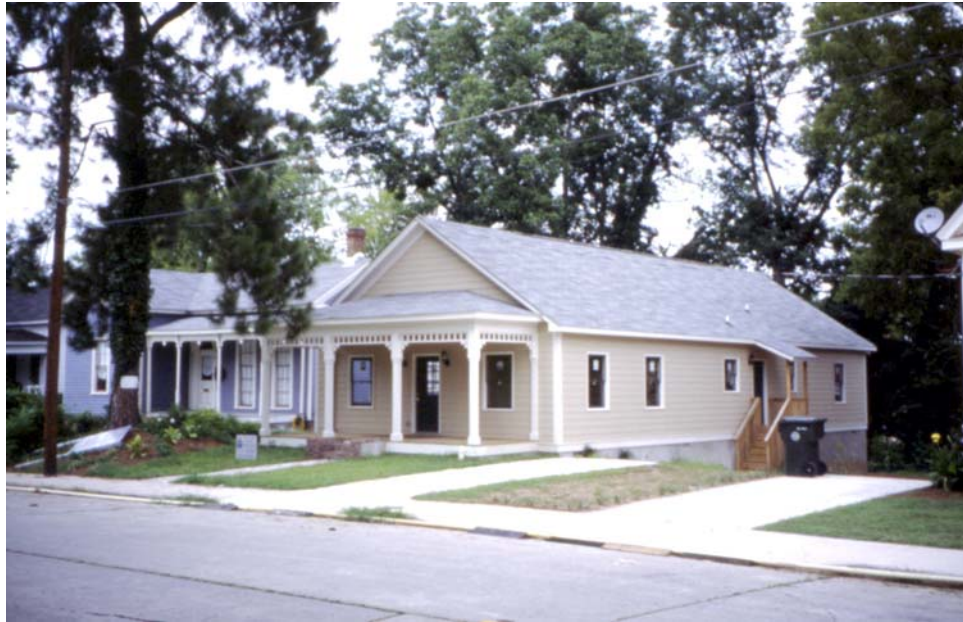
Figure 64: 1419 Chestnut Street After Infill. (Photograph by author, 2003)
