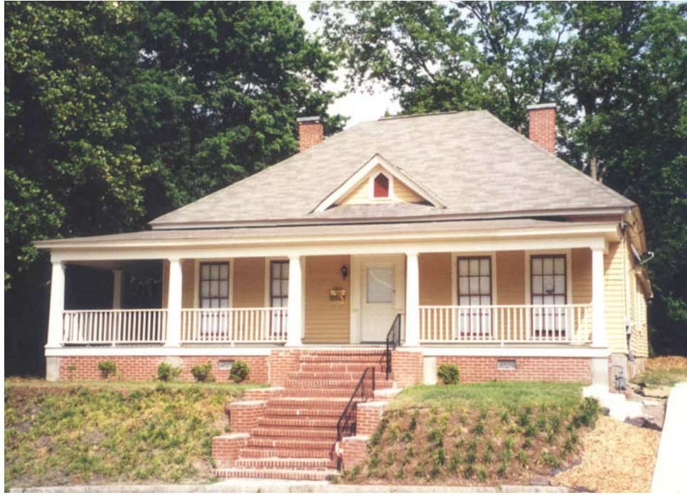
Figure 59: 842 Tatnall Street After Rehabilitation. (Photograph courtesy of Macon Heritage Foundation)
