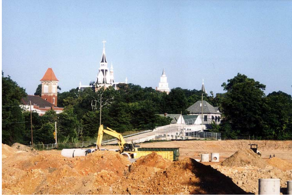
Figure 83: View of the Oglethorpe Homes Site After Demolition. (Photograph by author, 2003)
