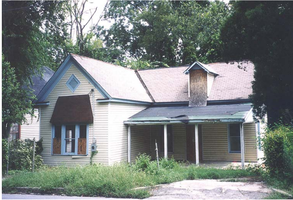
Figure 73: Vacant House at Ash and Ross Streets Identified for Demolition for Infill. (Photograph by author, 2003)
