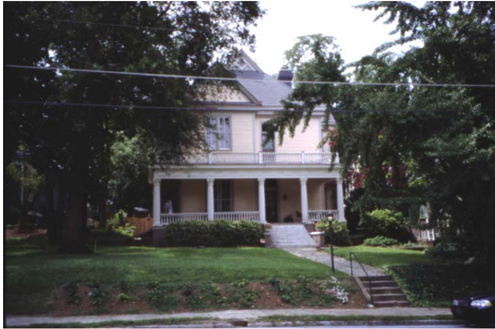
Figure 49: 1147 Adams Street After Rehabilitation. (Photograph by author, 2003)
