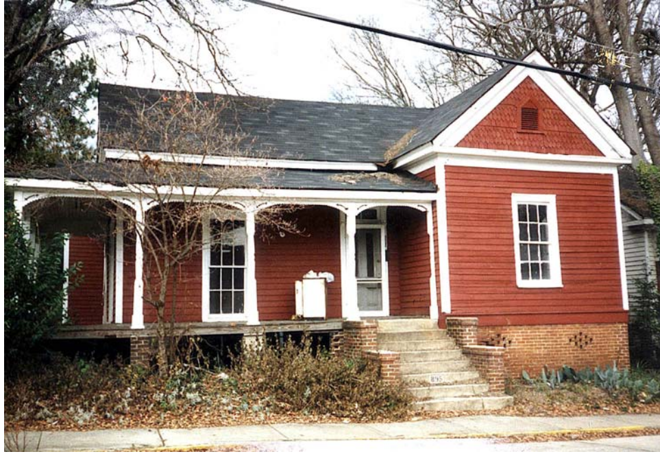
Figure 56: 895 Tatnall Street Before Rehabilitation. (Photograph by author, 2003)
