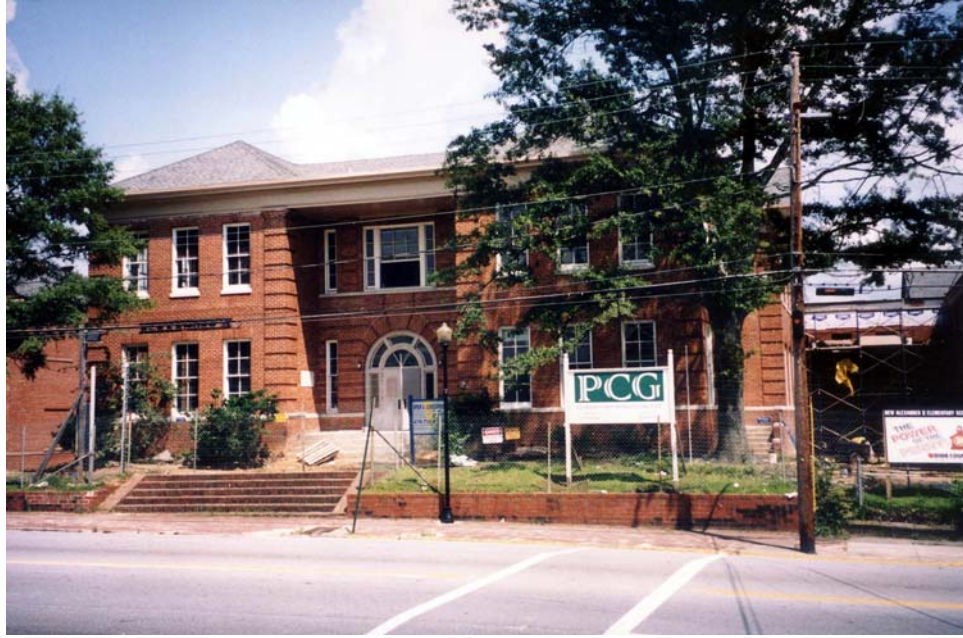
Figure 84: Historic Alexander II School Building During Rehabilitation (Photograph by author, 2003)
