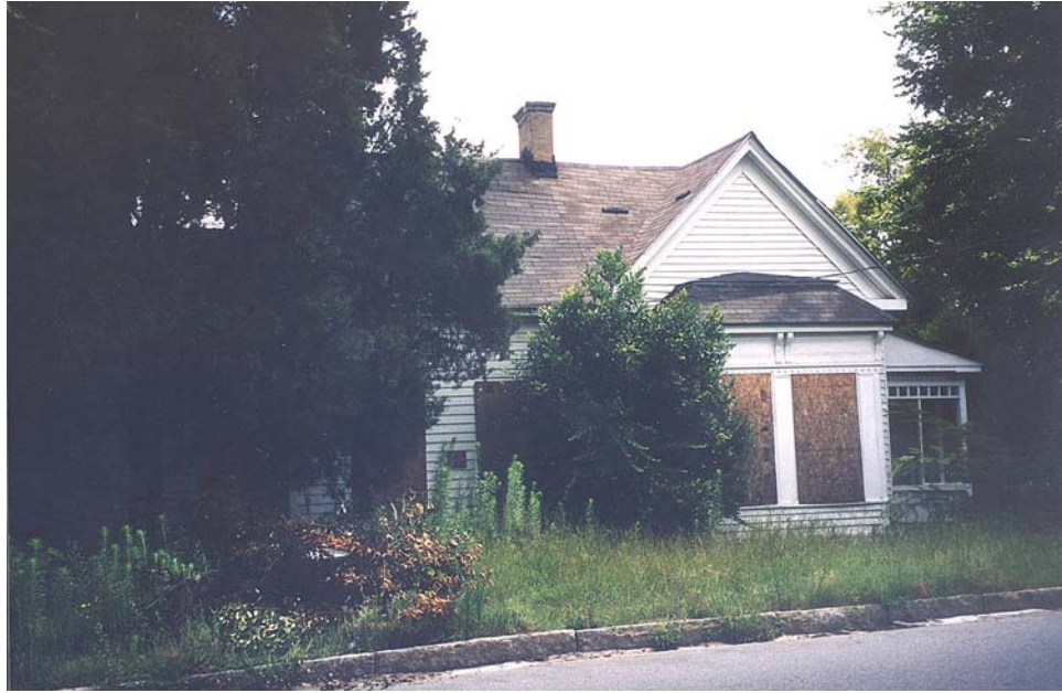
Figure 72: Vacant House at Ash and Ross Streets Identified for Rehabilitation. (Photograph by author, 2003)
