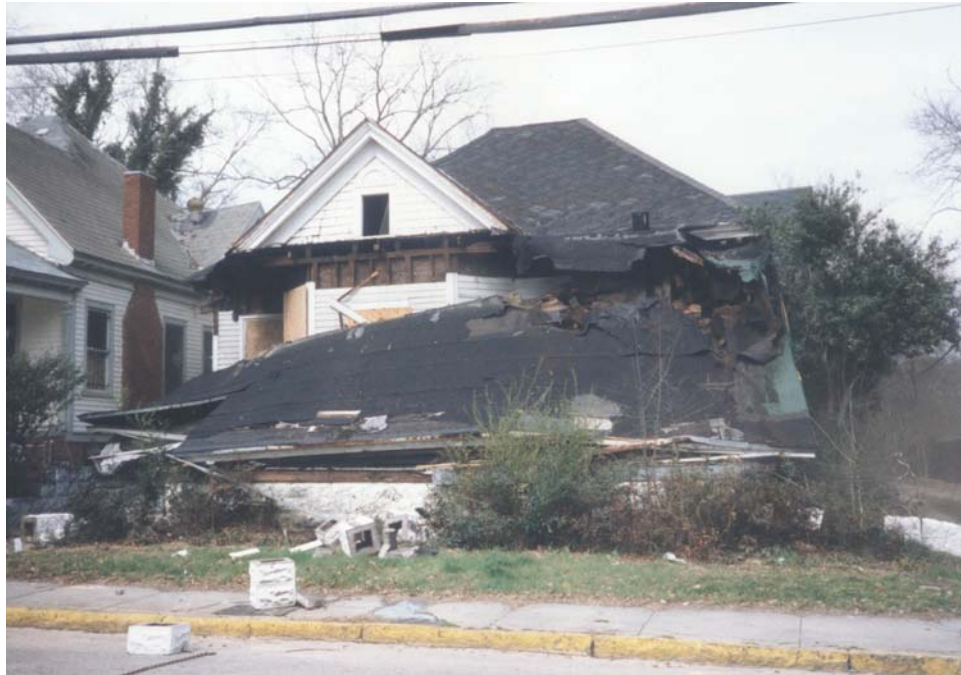
Figure 45: 1225 Linden Avenue Prior to Rehabilitation. (Photograph courtesy of Macon Heritage Foundation)
