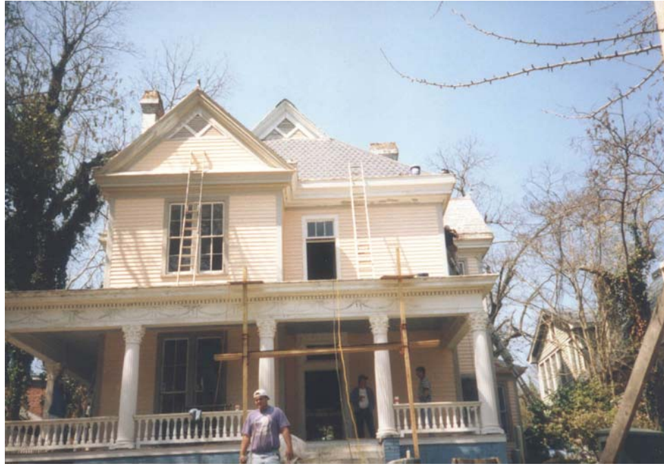
Figure 48: 1147 Adams Street During Rehabilitation. (Photograph courtesy of Macon Heritage Foundation)
