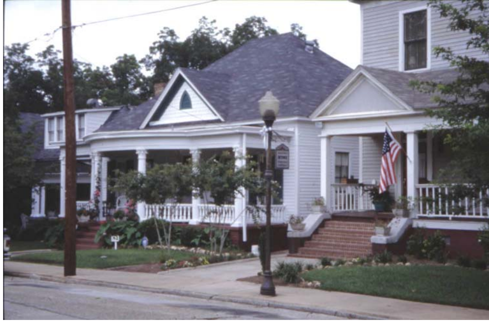
Figure 51: Private Rehabilitation at 1623 Lawton Avenue. (Photograph by author, 2003)
