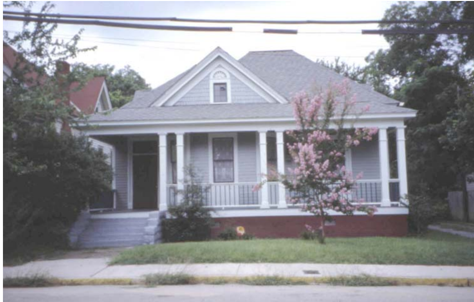
Figure 46: 1225 Linden Avenue After Rehabilitation. (Photograph by author, 2003)
