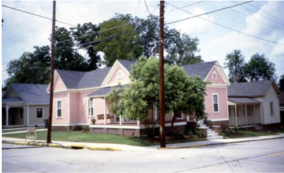
Figure 57: 895 Tatnall Street After Rehabilitation. (Photograph by author, 2003)
