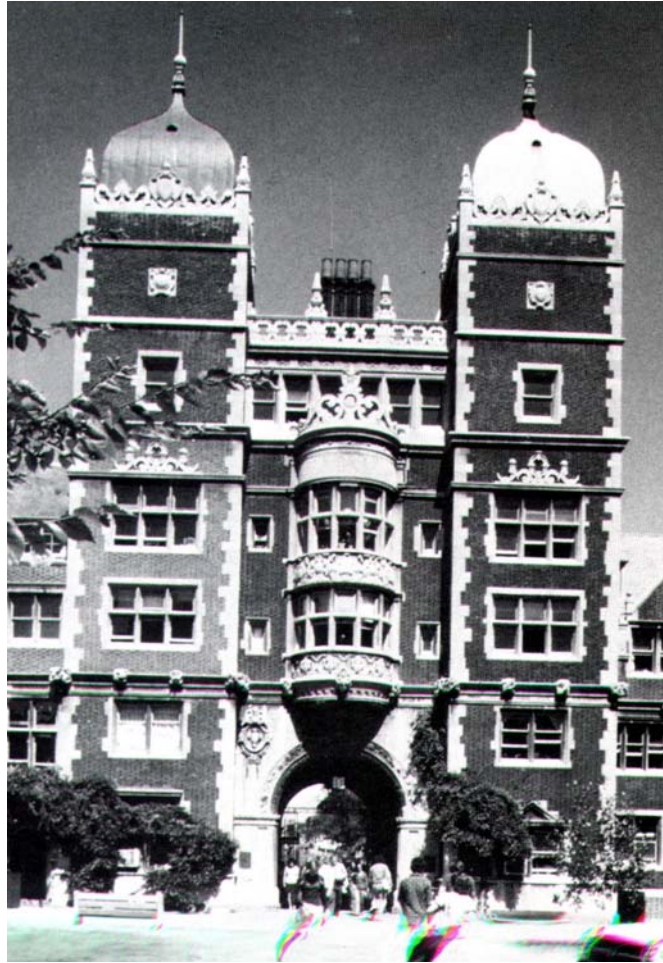
Figure 33: Memorial Gateway Tower in Residence Hall Designed by Cope and Stewardson. Photograph by Buford Pickens. (Paul Venable Turner, Campus: An American Planning Tradition , Cambridge, Massachusetts, 1984, p. 225)
