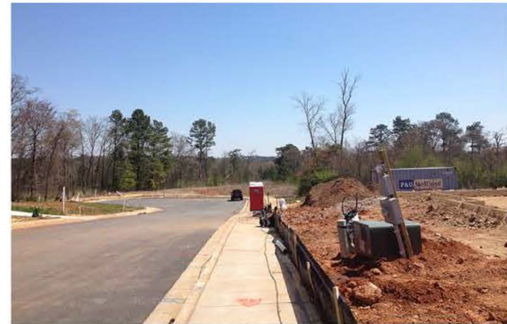
Sidewalk adjacent to Phase II, facing end of cul-de-sac
