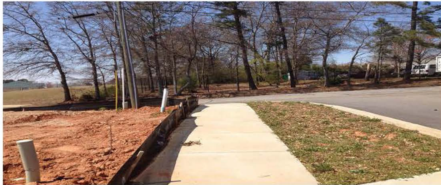
Sidewalk adjacent to Phase II, facing Bray St.
