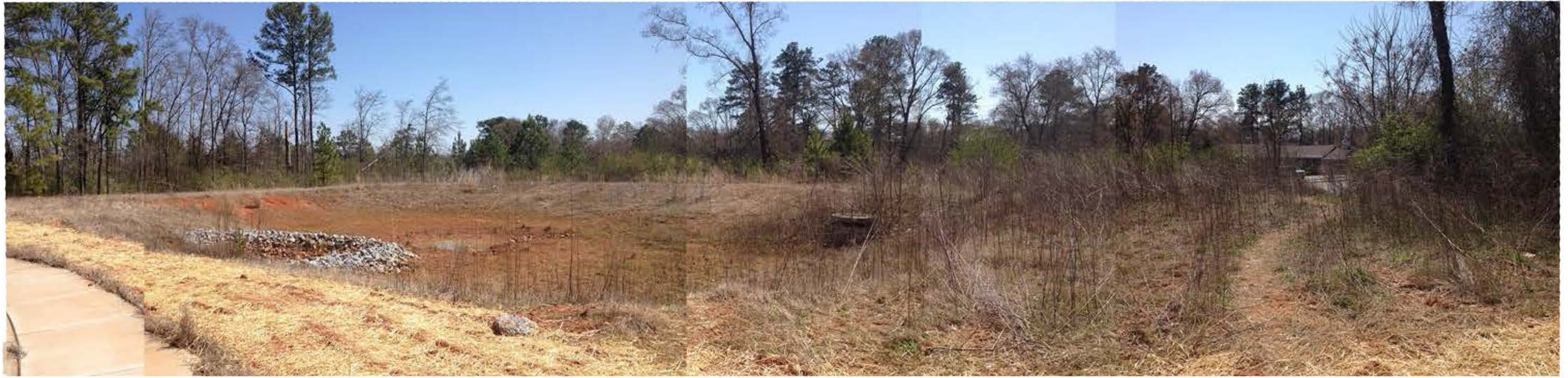
View of Stormwater Detention Pond
