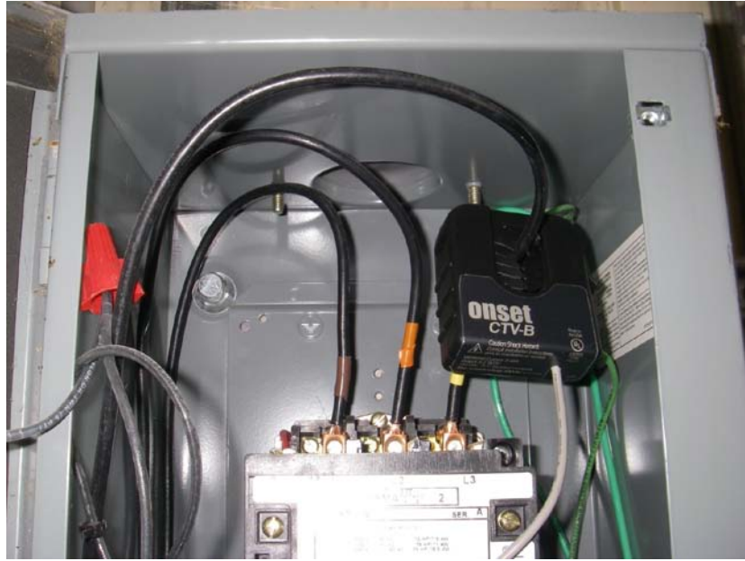
Figure 4.1: A current sensor (top right) installed on a pump at the pasture-based dairy.
