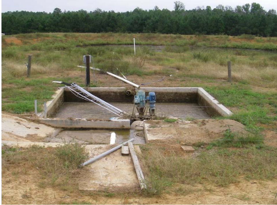
Figure 5.1: From the foreground: the sand-trap, storage tank and pump, and overflow lagoon.
