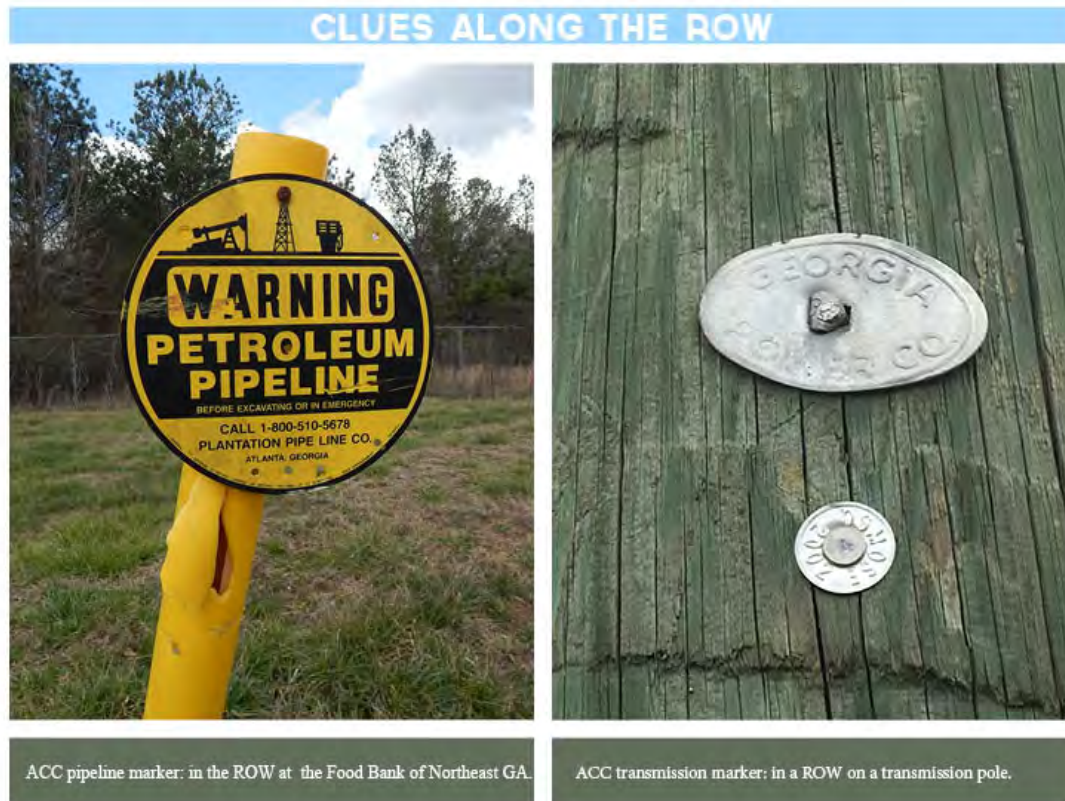
Figure 2.2: Pipeline & Transmission Pole Markers in ACC ROWS Photo credit: Elizabeth Beak
