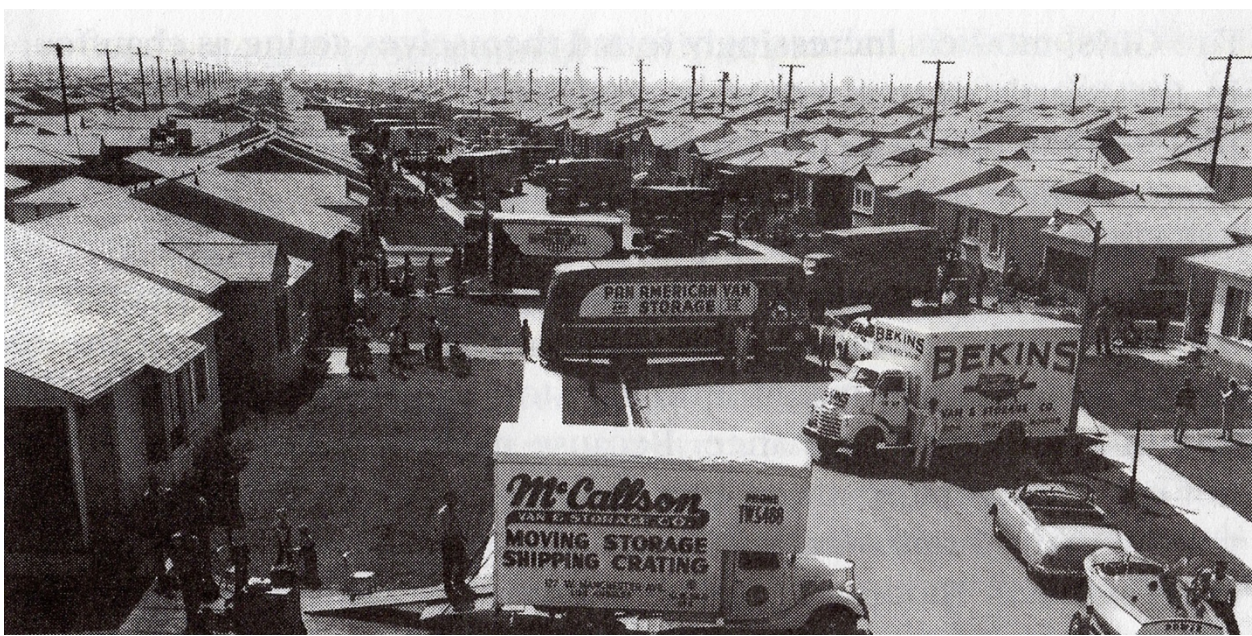
Figure 14. Families moving into newly constructed suburban homes in Van Nuys, California.
