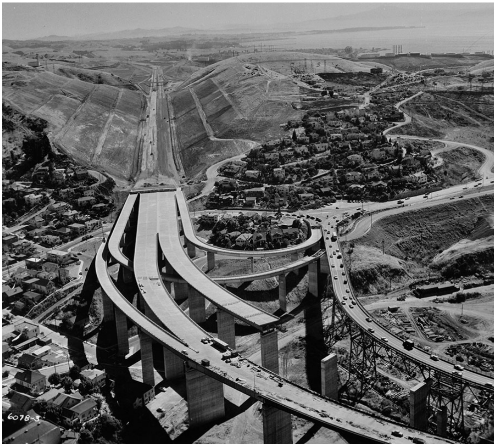
Figure 13. Construction of a highway interchange.
