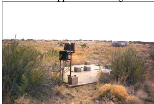
Concrete support for cooling tank
