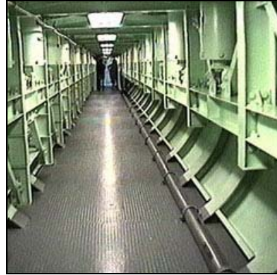
Fig. 4-4: Restored cableway connecting launch complex and silo chamber (Walton 1998)
