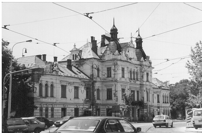
Figure 70 The abandoned and dilapidated Vyšehradské nádraží , or Vyšehrad railway station, built at the turn of the nineteenth and twentieth centuries; photo taken by author in June 2000 and in her possession.
