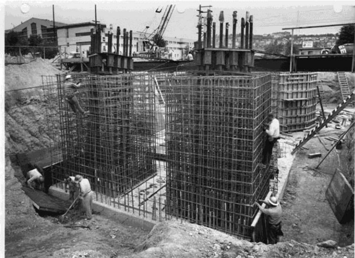
Figure 6: Image 2005.6.9, Robert Dudley, Space Needle Foundation Under Construction, June 6, 1961, Museum of History and Industry Photograph Collection, University of Washington Libraries, Special Collections Division
