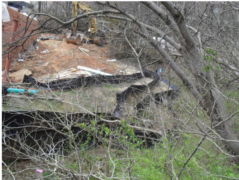
Figure 82: Erosion control from University of Tennessee construction site on the banks of Lower Second Creek
