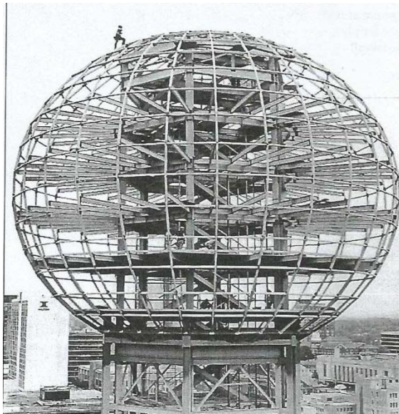
Figure 72: Construction of SunSphere, from Knoxville's 1982 World's Fair , 96.
