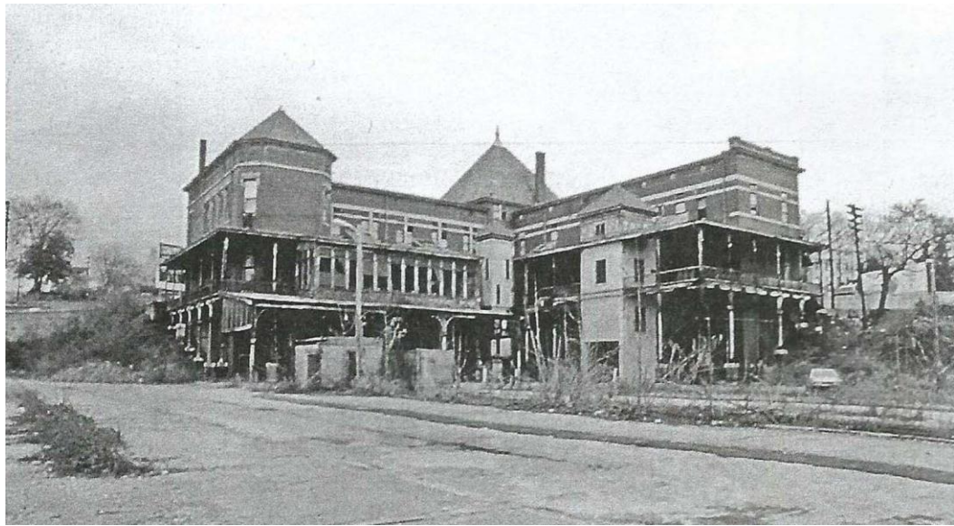
Figure 36: L&N Depot (built in 1917) before restoration for Energy Expo '82, from Knoxville's 1982 World's Fair , 13.
