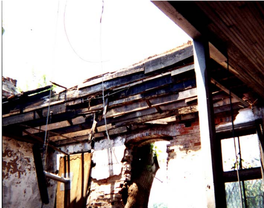
Figure 13. Cottonwood tree growing through the rear façade of the Fitzpatrick Hotel (2002)
