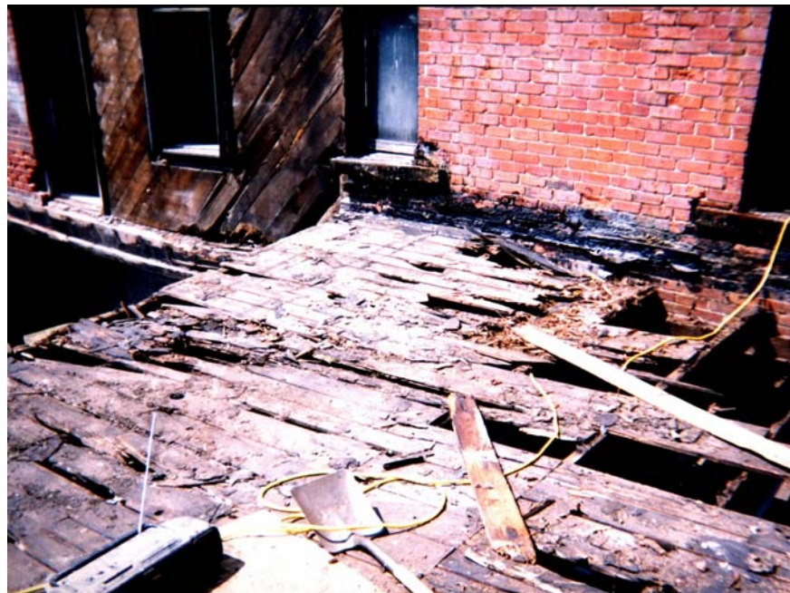
Figure 12. Pre-rehabilitation water damage in the Fitzpatrick Hotel (2002)
