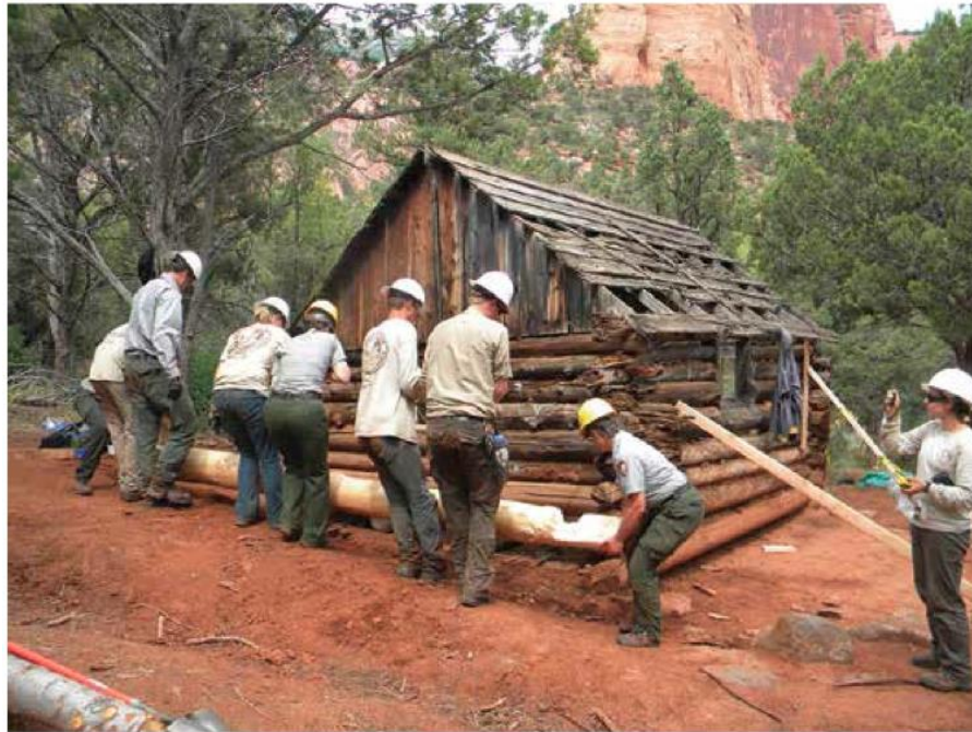
Figure 12: Zion National Park staff rehabilitating historic cabin located in wilderness, Zion National Park 376
