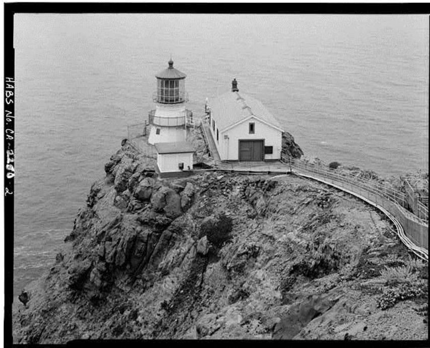
Figure 3: Point Reyes Lighthouse, Point Reyes National Seashore 200
