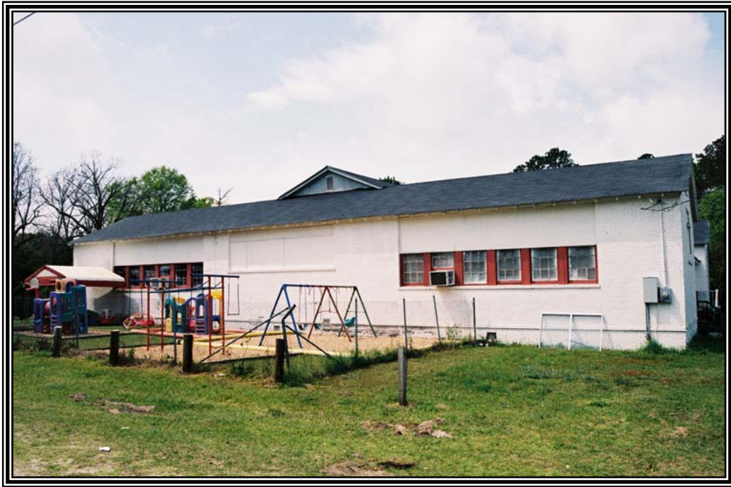
View of the east side elevation of the former Camilla Colored School facing southwest from the west side of North Ellis Street.
