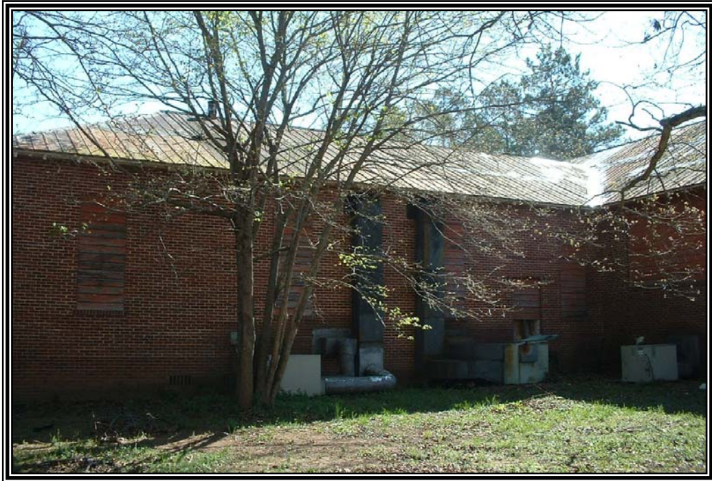
View of the rear of the former Teacher Training and Industrial School facing southeast from the north side of Danielsville Road.
