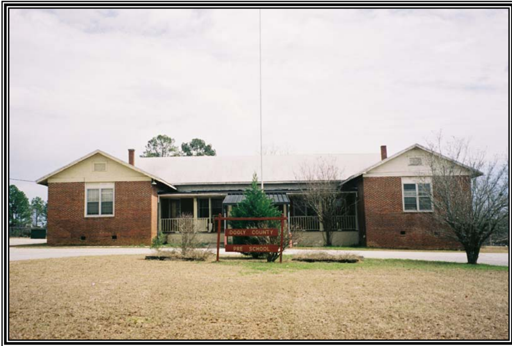
View of façade of the former Vienna High and Industrial School facing east from the east side of 9 th Street.
