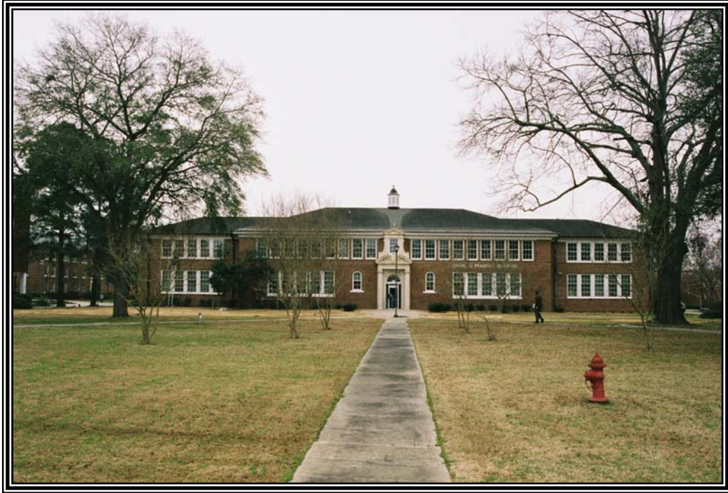
View of Davison Hall Dormitory in Fort Valley State College Historic District facing northwest from campus quadrangle.
