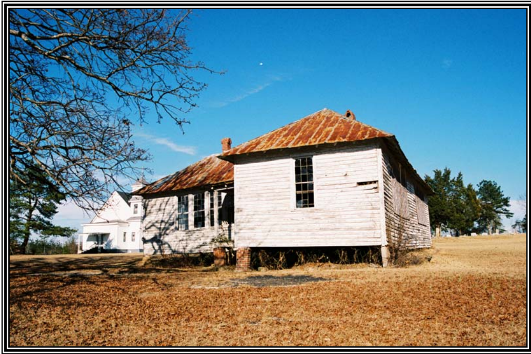
View of the west side elevation of the former Hickory Grove School facing east from the east side of Hickory Grove Church Road.
