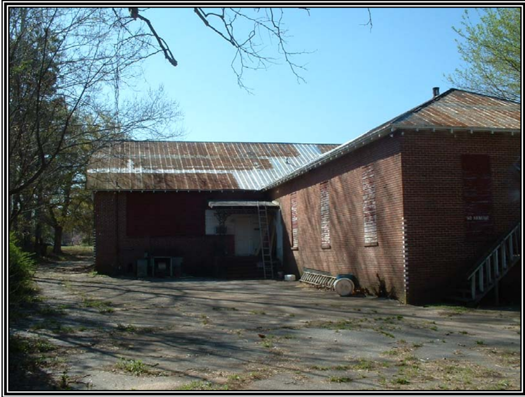
View of the rear of the former Teacher Training and Industrial School facing south from the north side of Danielsville Road.
