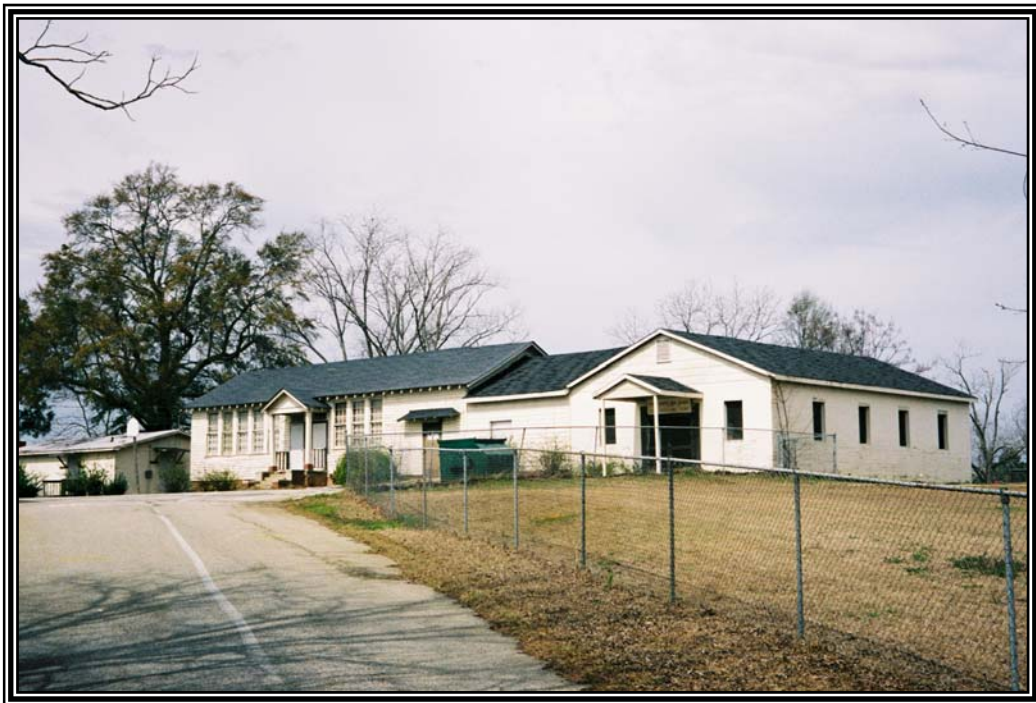
Oblique view of façade and east side elevation of secondary building on the grounds of the former Vienna High and Industrial School facing northwest from the west side of State Route 27.
