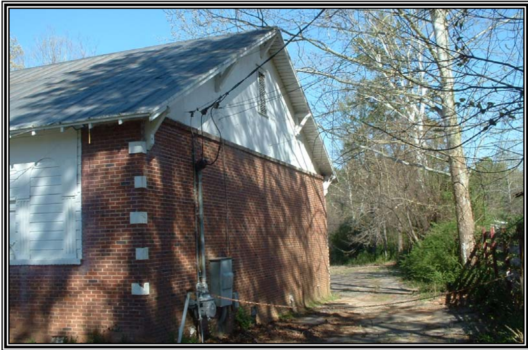
View of the east side elevation of the former Teacher Training and Industrial School facing northwest from the north side of Danielsville Road.
