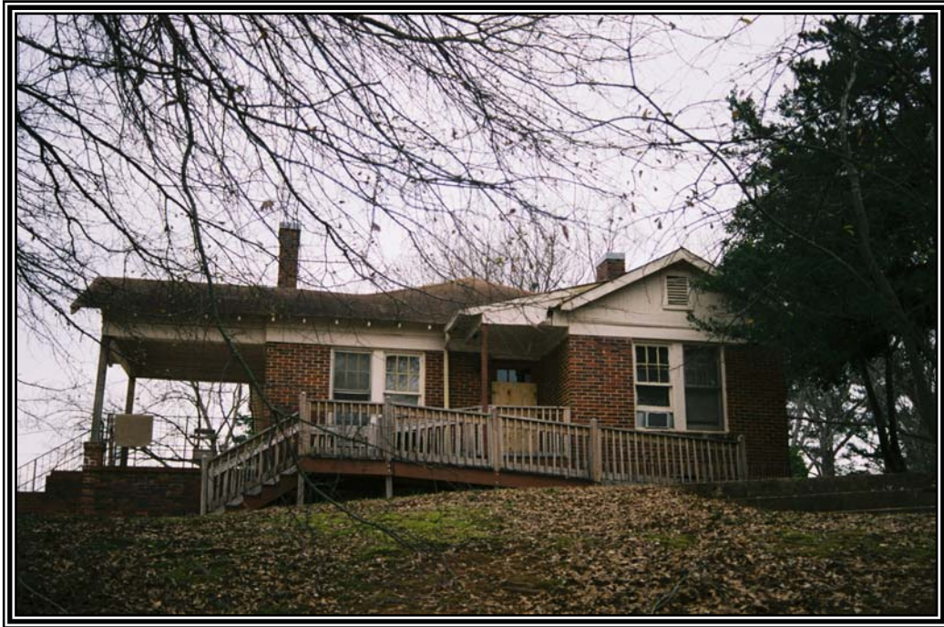
View of façade of Teachers' Cottage facing north from the north side of Washington Drive.
