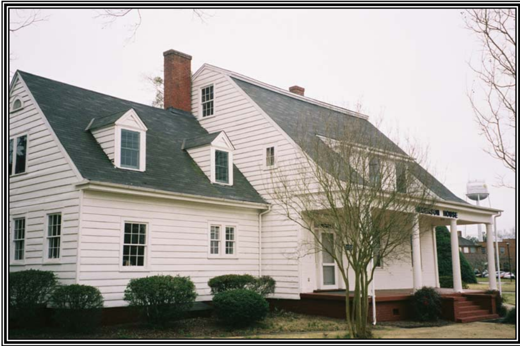
View of Anderson House in Fort Valley State College Historic District facing south from south side of State University Drive.
