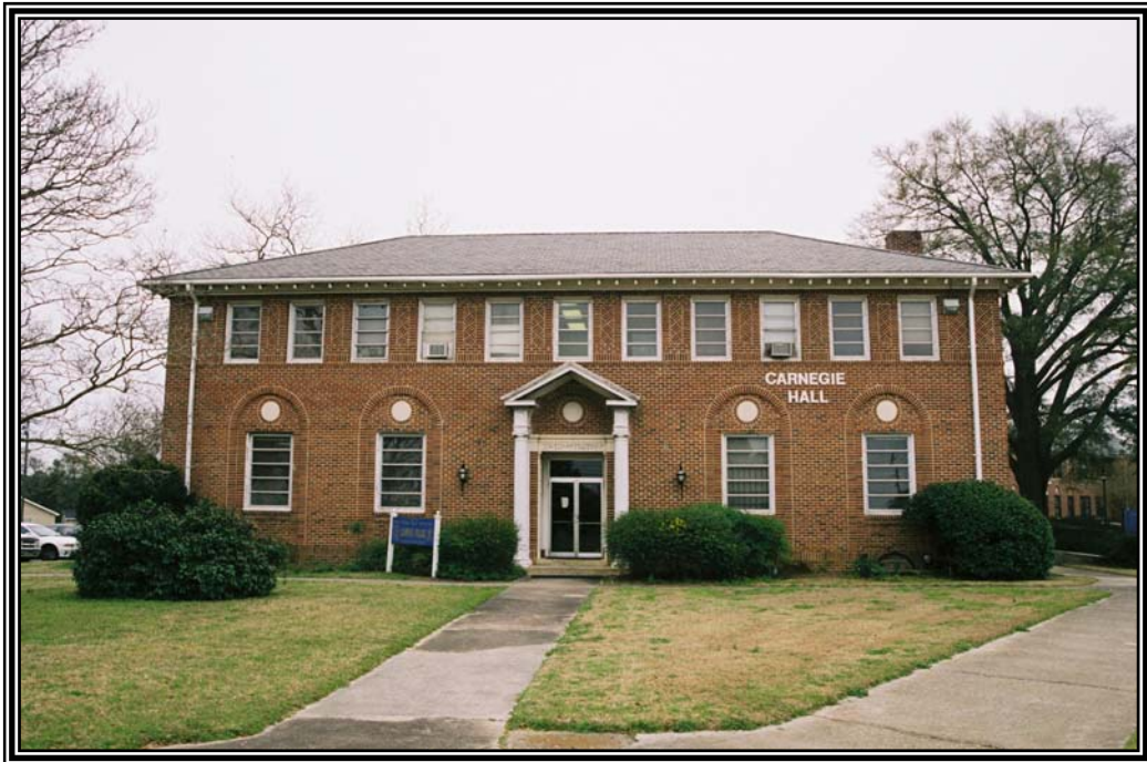
View of Carnegie Hall in Fort Valley State College Historic District facing south from south side of State University Drive.
