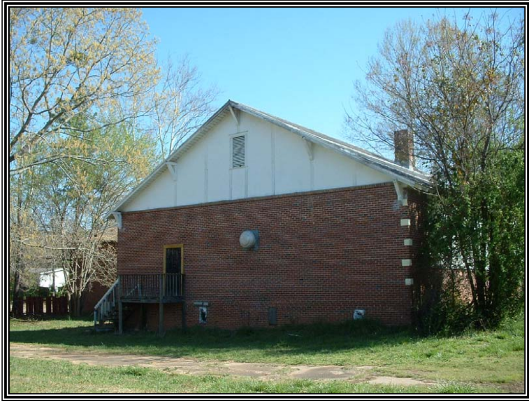
View of the west side elevation of the former Teacher Training and Industrial School facing northeast from the north side of Danielsville Road.
