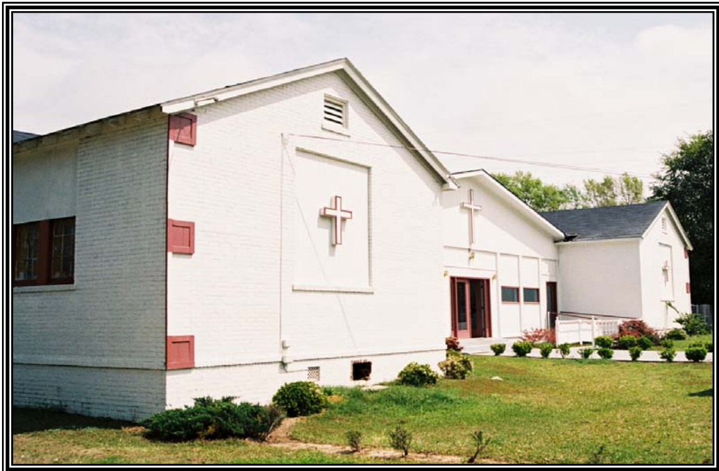
Oblique view of the façade of the former Camilla Colored School facing northeast from the north side of Thompson Street.
