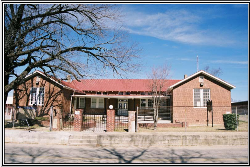
View of façade of the former Thomas Jefferson Elder High and Industrial School facing north from the south side of Hall Street.
