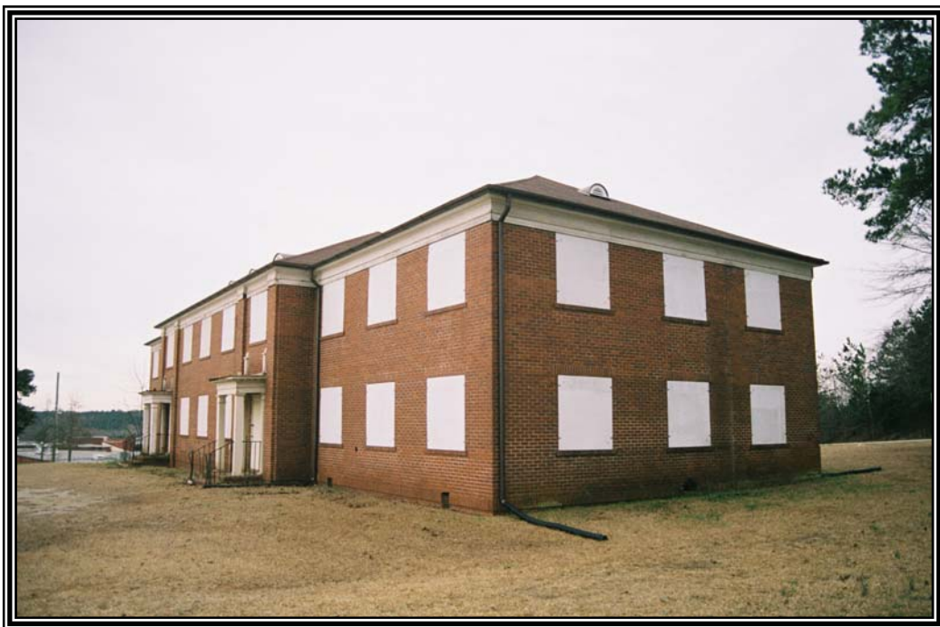
Oblique view of façade and east side elevation of Women's Dormitory northwest from the east side of State Route 83.
