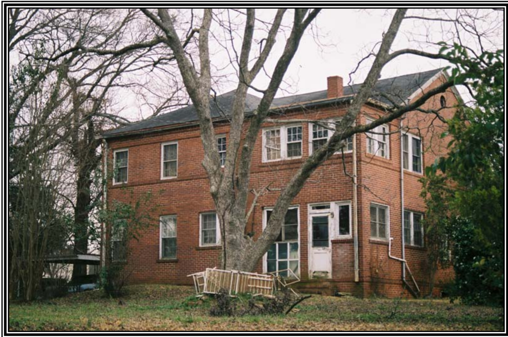
View of rear and side elevations of President's House (not included in National Register listing at property owner's request) facing southeast from north side of Washington Drive.
