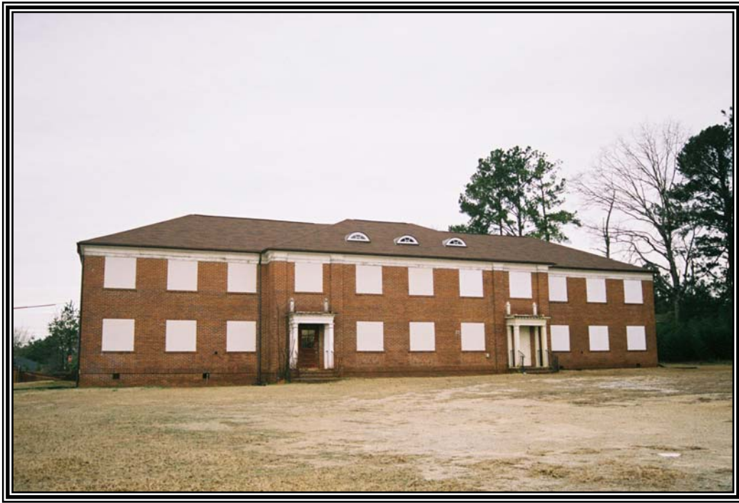
View of façade of State Teachers and Agricultural College for Negroes Women's Dormitory facing northwest from the east side of State Route 83.
