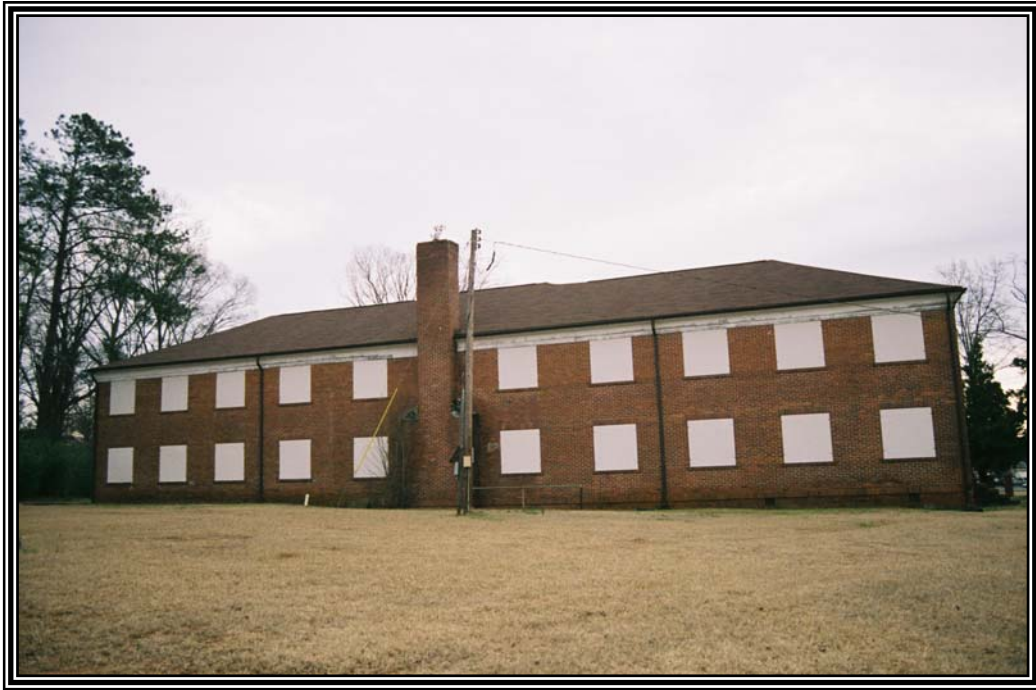
View of rear elevation of Women's Dormitory facing south from the south side of State Route 83.
