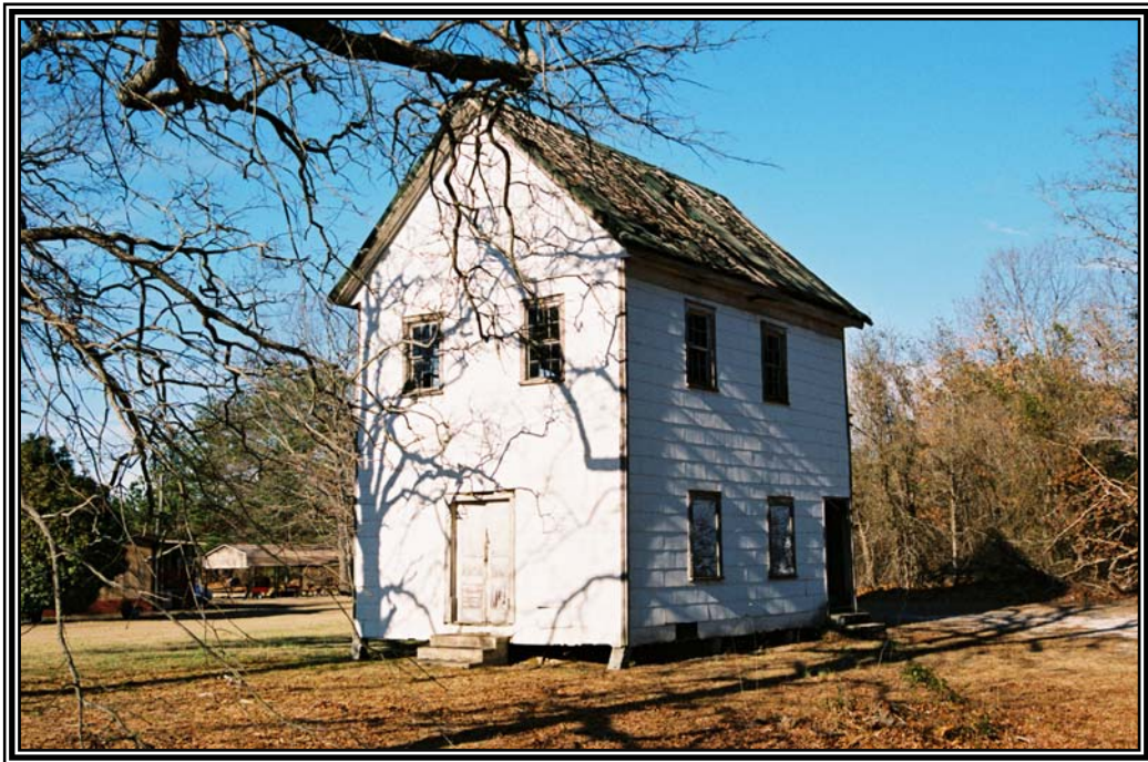
Oblique view of the façade and south side elevation of apparent dormitory of the former Hickory Grove School facing northeast from the east side of Hickory Grove Church Road.
