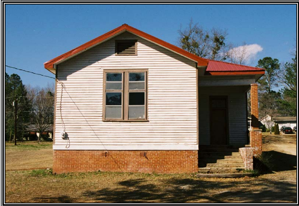
View of façade of the former Hiram Colored School facing north from the west side of State Route 92.
