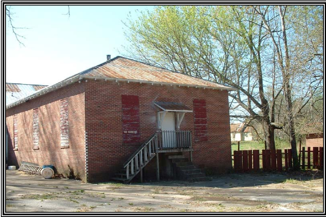
View of the rear of the former Teacher Training and Industrial School facing southwest from the north side of Danielsville Road.
