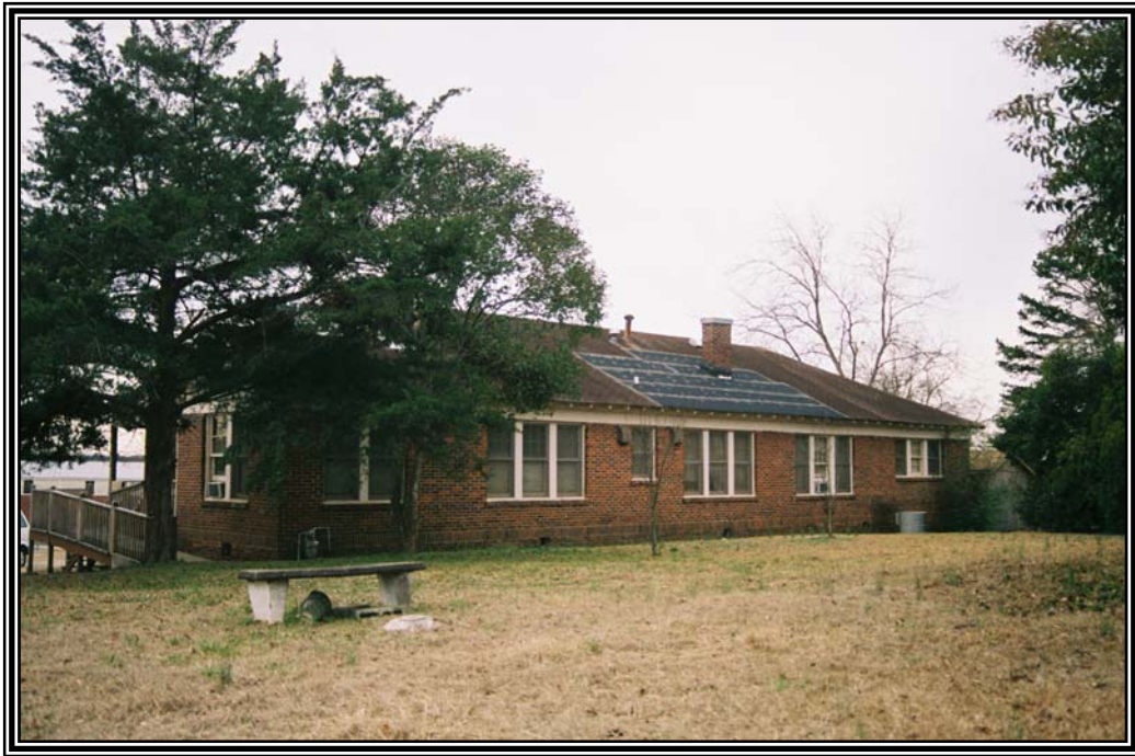
View of east side elevation of Teachers' Cottage facing northwest from the north side of Washington Drive.
