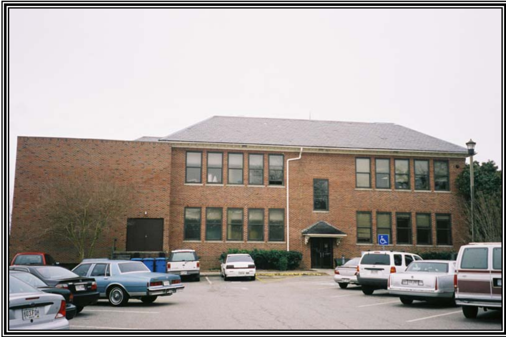
View of east side elevation of Founders Hall (former F.V.H.I.S. Academic Building) facing west from south of the campus quadrangle.
