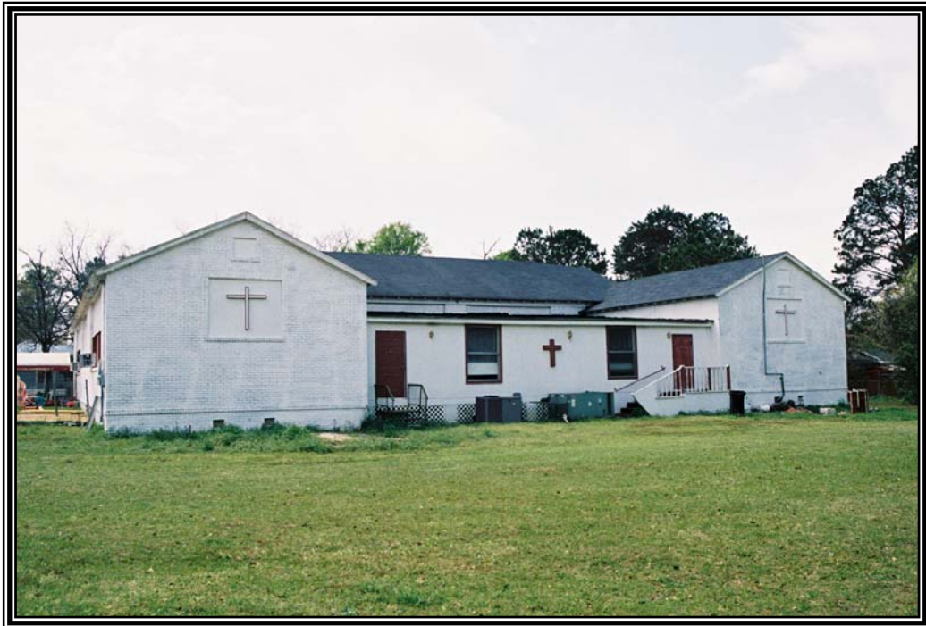
View of the rear elevation of the former Camilla Colored School facing south from the south side of Cemetery Road.
