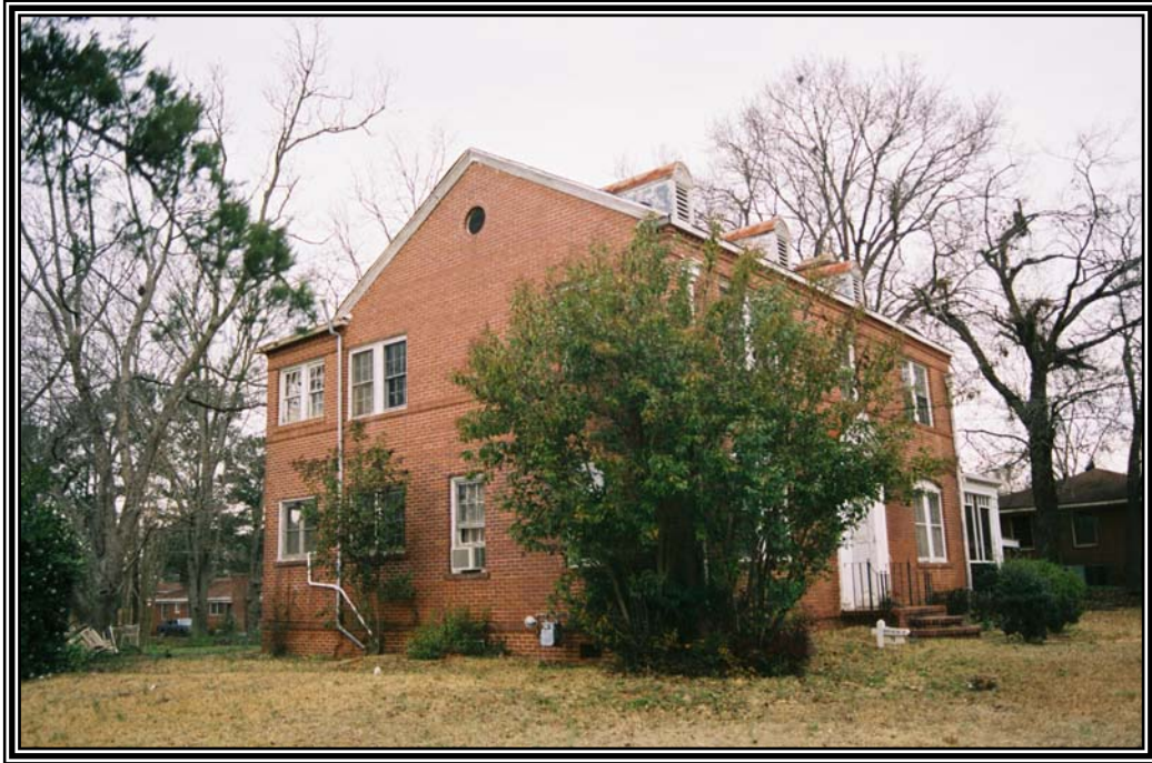
Oblique view of façade and west side elevation of President's House (not included in National Register listing at property owner's request) facing northeast from north side of Washington Drive.
