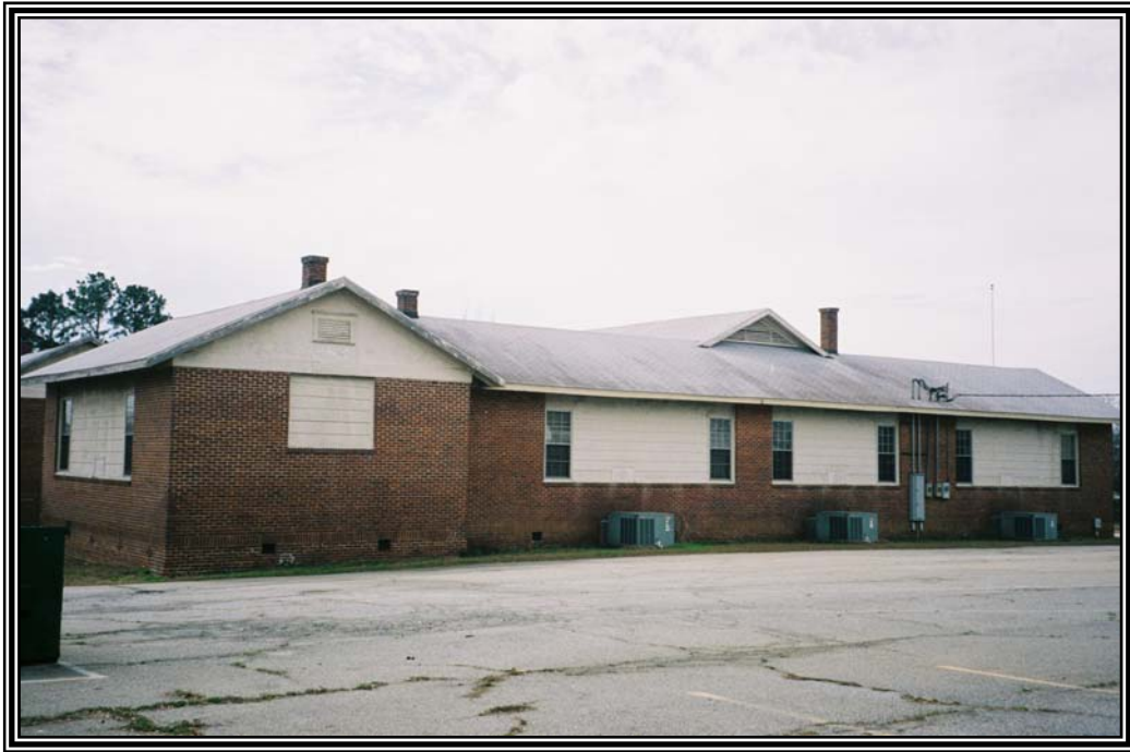
Oblique view of the north side elevation of the former Vienna High and Industrial School facing southwest from the west side of State Route 27.
