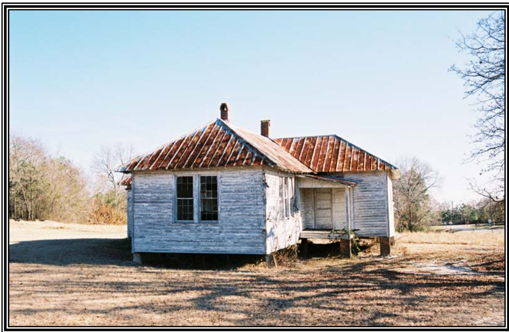
View of the rear elevation of the former Hickory Grove School facing northwest from the east side of Hickory Grove Church Road.
