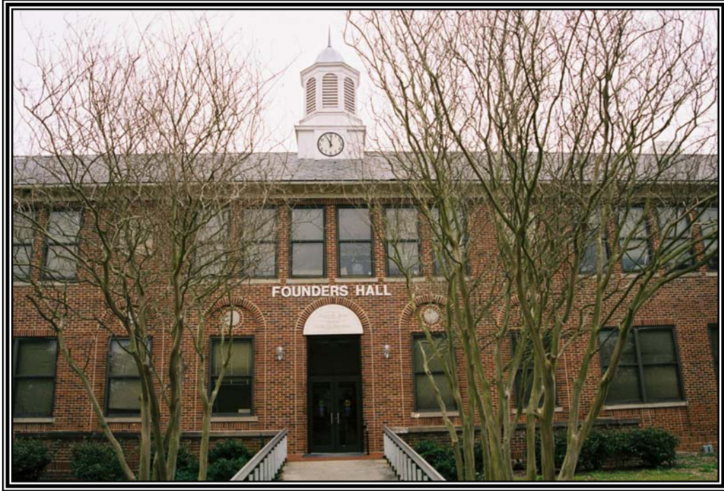
View of façade of Founders Hall (former F.V.H.I.S. Academic Building) facing southeast from campus quadrangle.
