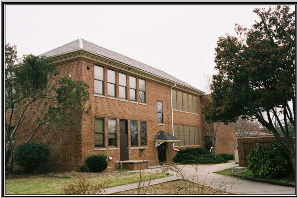
Oblique view of west side elevation of Founders Hall (former F.V.H.I.S. Academic Building) facing southeast from the campus quadrangle.
