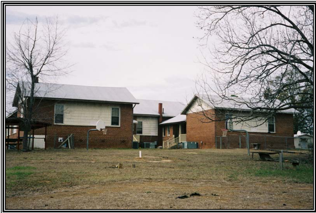
View of the rear elevation of the former Vienna High and Industrial School facing west from the west side of State Route 27.
