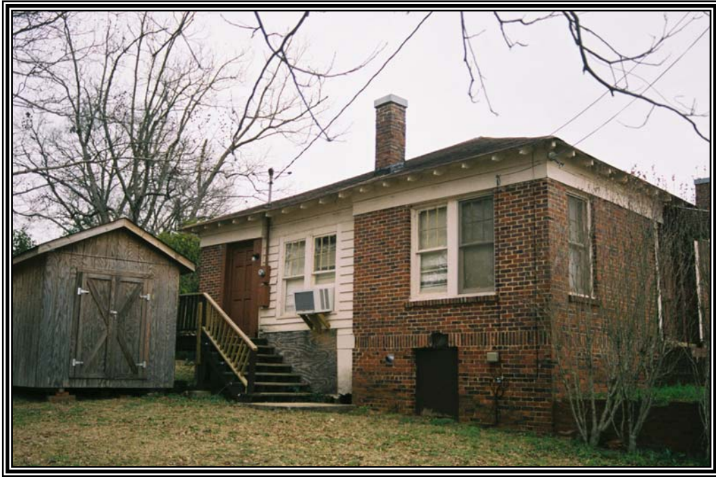
Oblique view of rear elevation of Teachers' Cottage facing southeast from the north side of Washington Drive.
