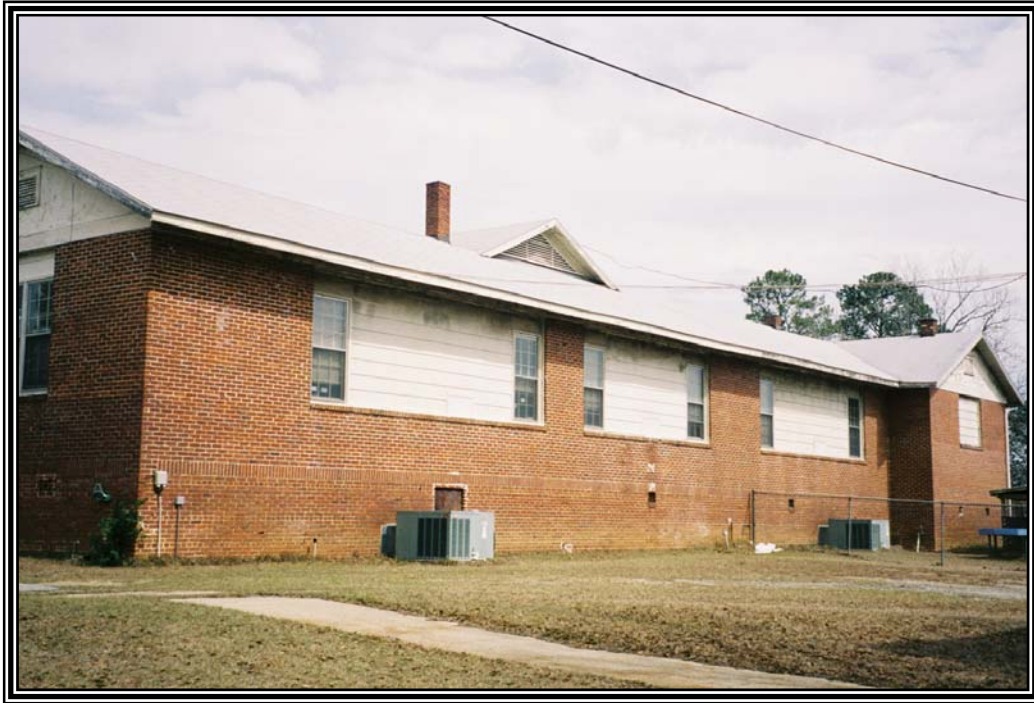
Oblique view of the south side elevation of the former Vienna High and Industrial School facing northeast from the east side of 9 th Street.
