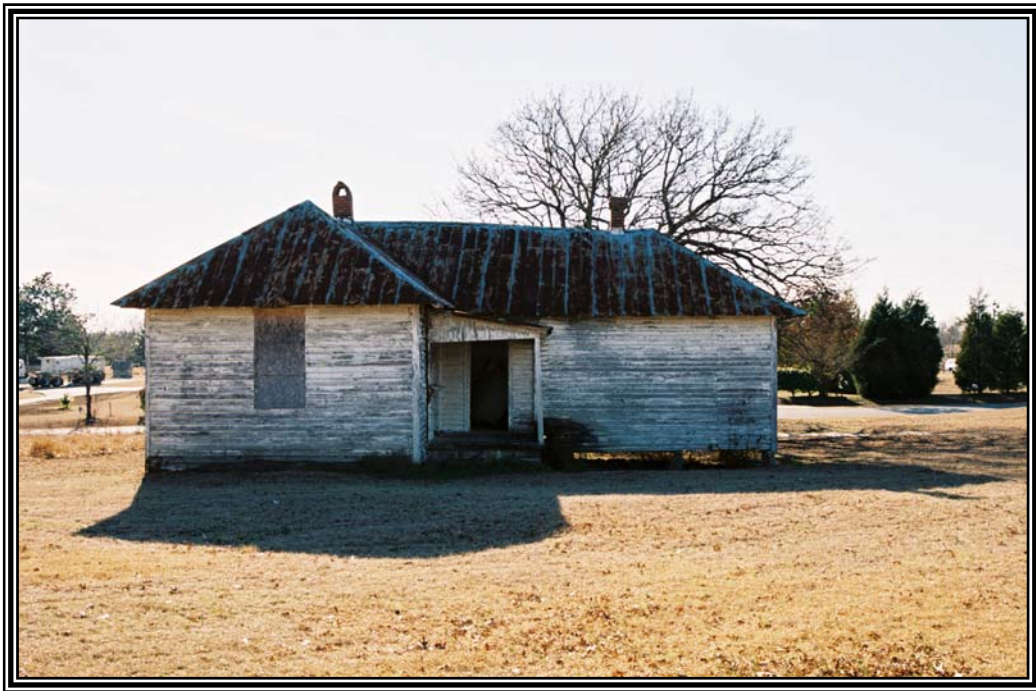
View of the east side elevation of the former Hickory Grove School facing southwest from the east side of Hickory Grove Church Road.
