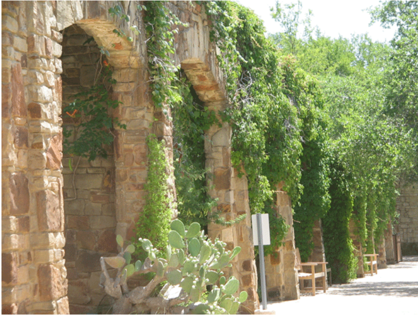
Figure 3.12 - Aqueduct leading from the auditorium roof to the cistern in the entrance garden 81
