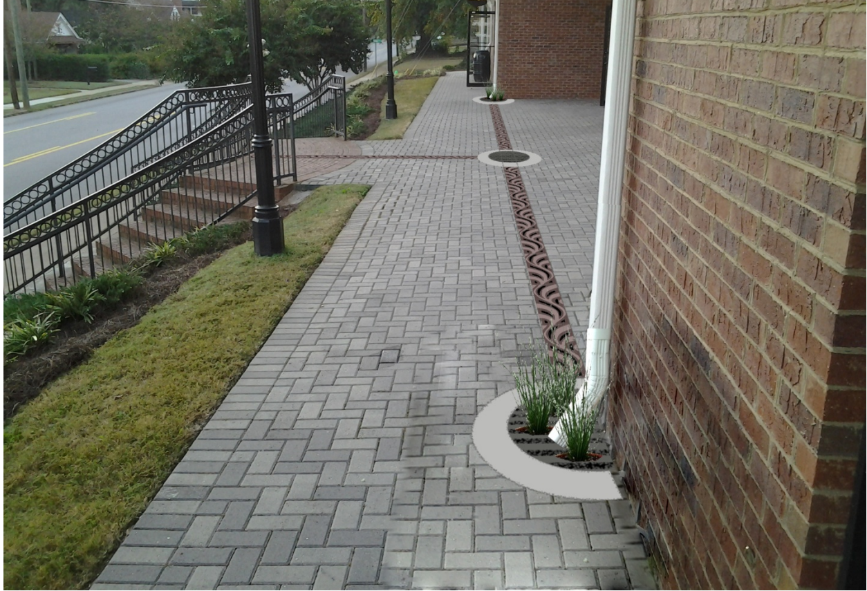
Figure 5.16 - Articulated drainage at front of Hodgson Terrace leading to hemicircular basin below
