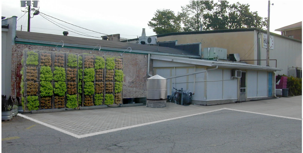
Figure 5.9 - Cistern and green wall next to Five & Ten
