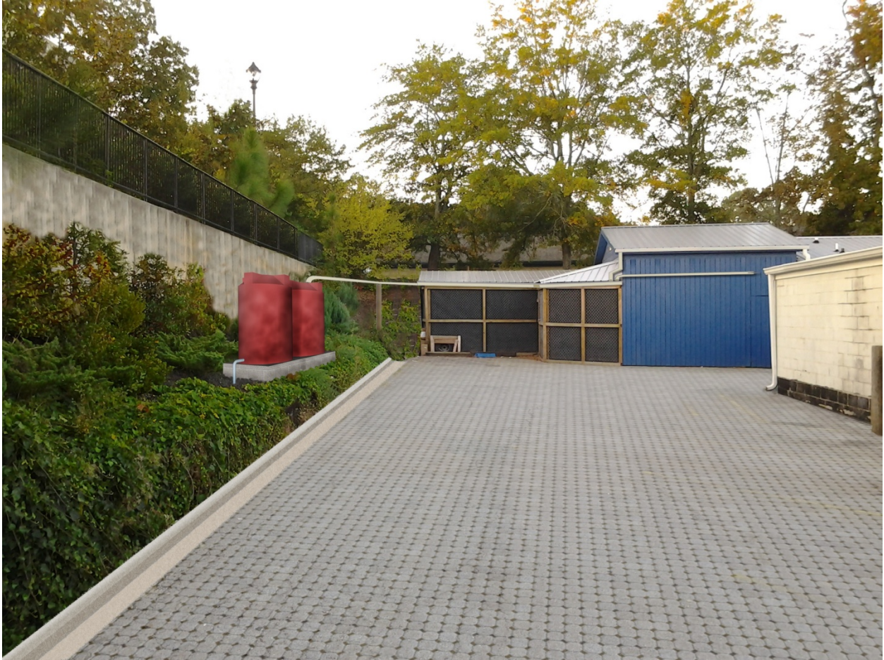
Figure 5.14 - Bottle Shop Extension rainwater stored by cisterns for use on terrace
