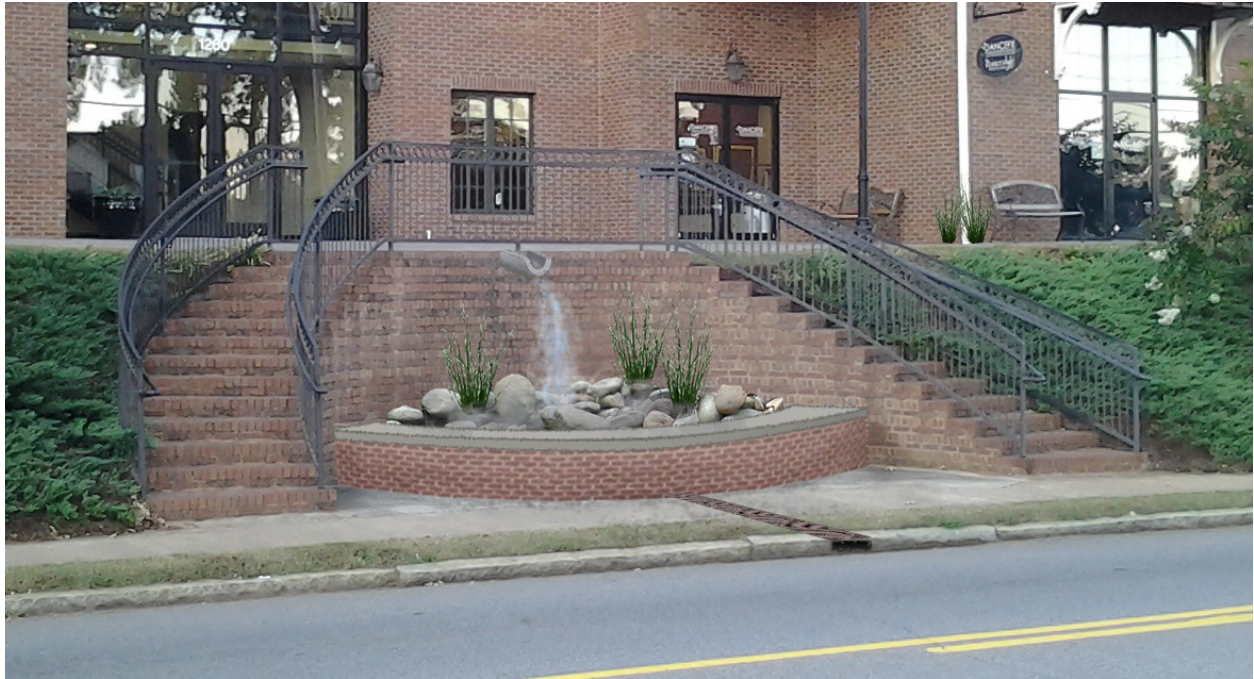
Figure 5.17 - Hemicircular basin with delayed drainage to street and drip irrigation to slope
