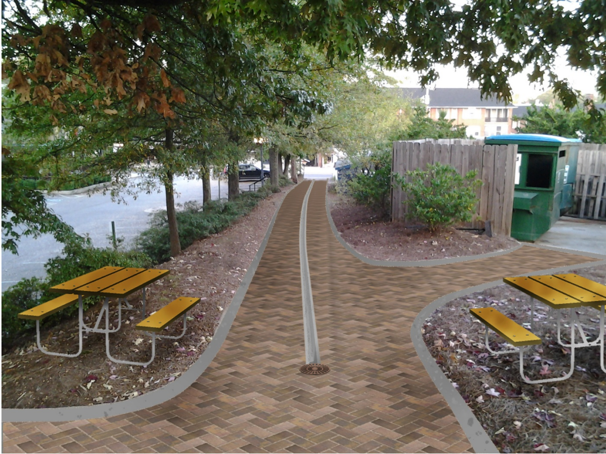
Figure 5.20 - Public alley rill, starting at peak elevation of path
