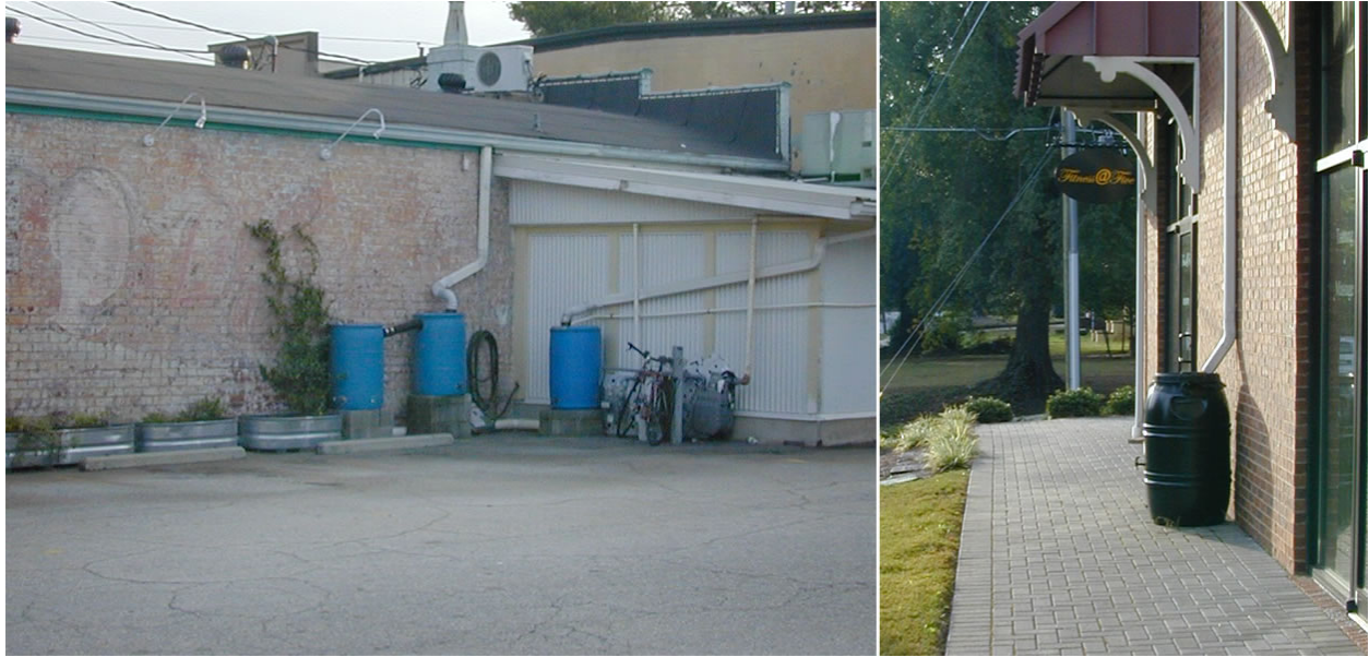
Figure 5.4 - Existing rain barrels
