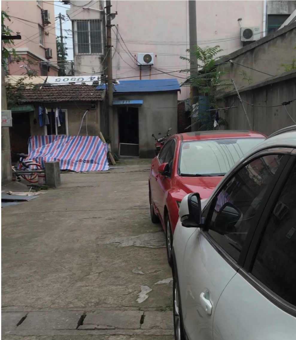
Figure 103: The illegal structures on the site (photo by author)
