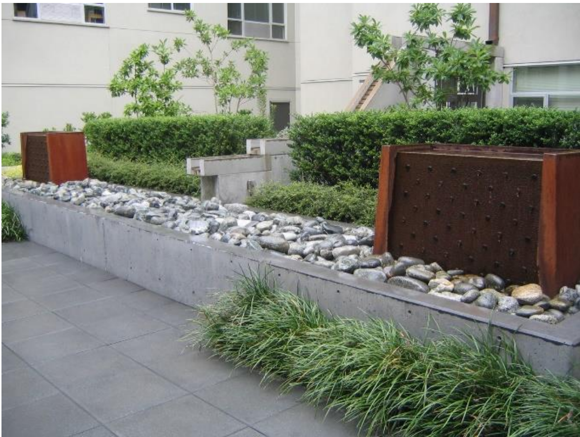
Figure 45: Two Corten weir boxes in 10th@Hoyt (Echols and Pennypacker 2015)
