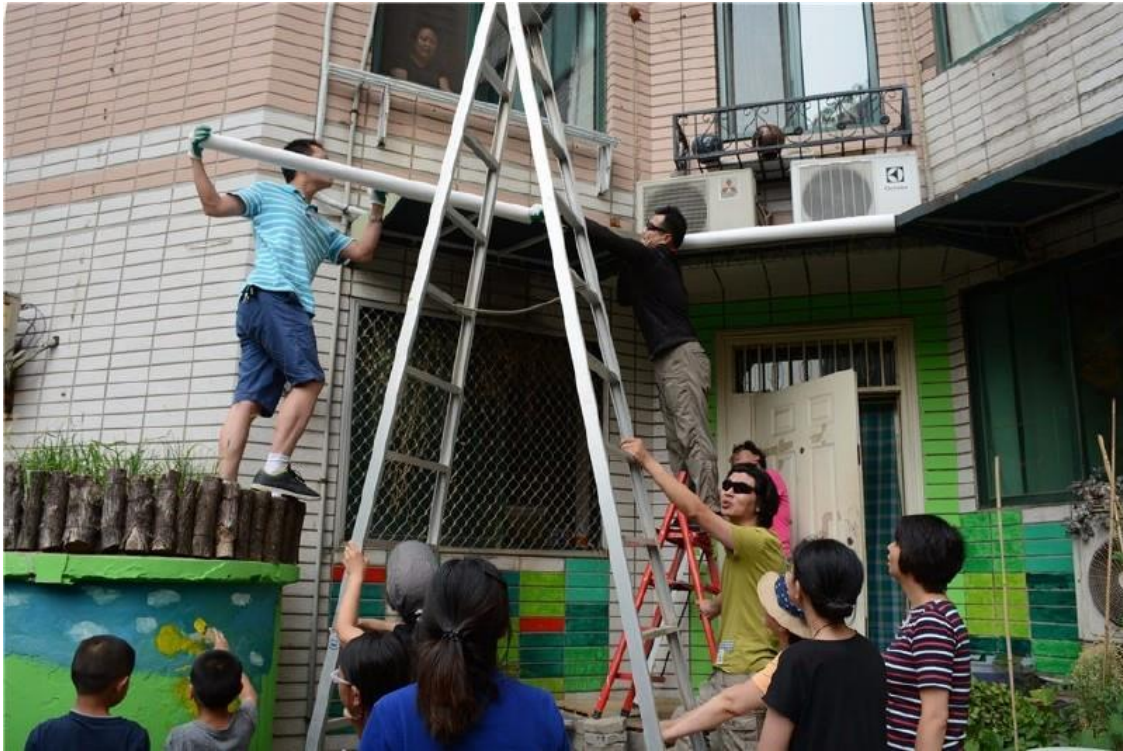
Figure 6: Residents help build the rainwater harvesting system
