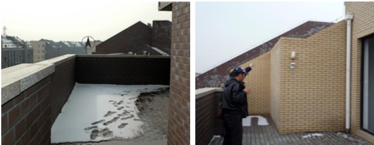
Figure 25: The balcony before transformation (Yu 2016)
