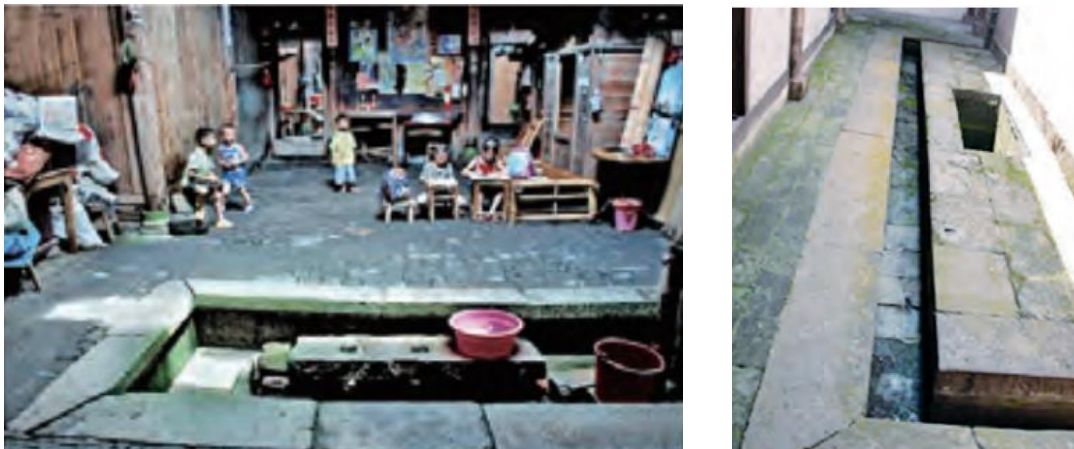
Figure 9: Drainage channel in the center of Tianjing (Wei and Wang 2016)
