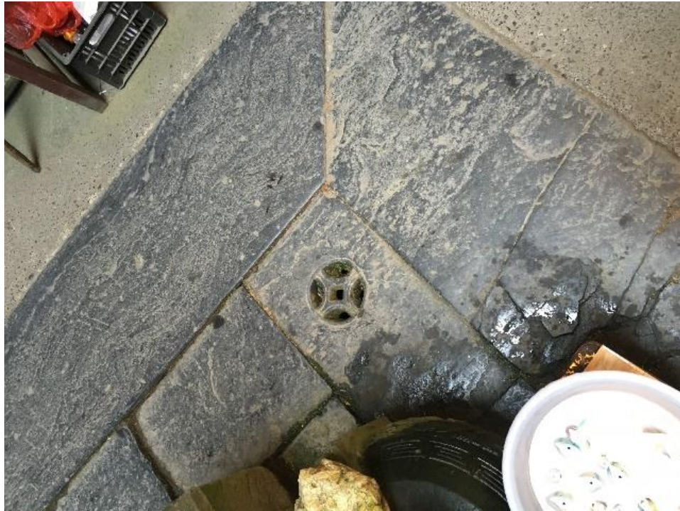
Figure 8: Picture of drainage hole in Tianjing (photo by author)
