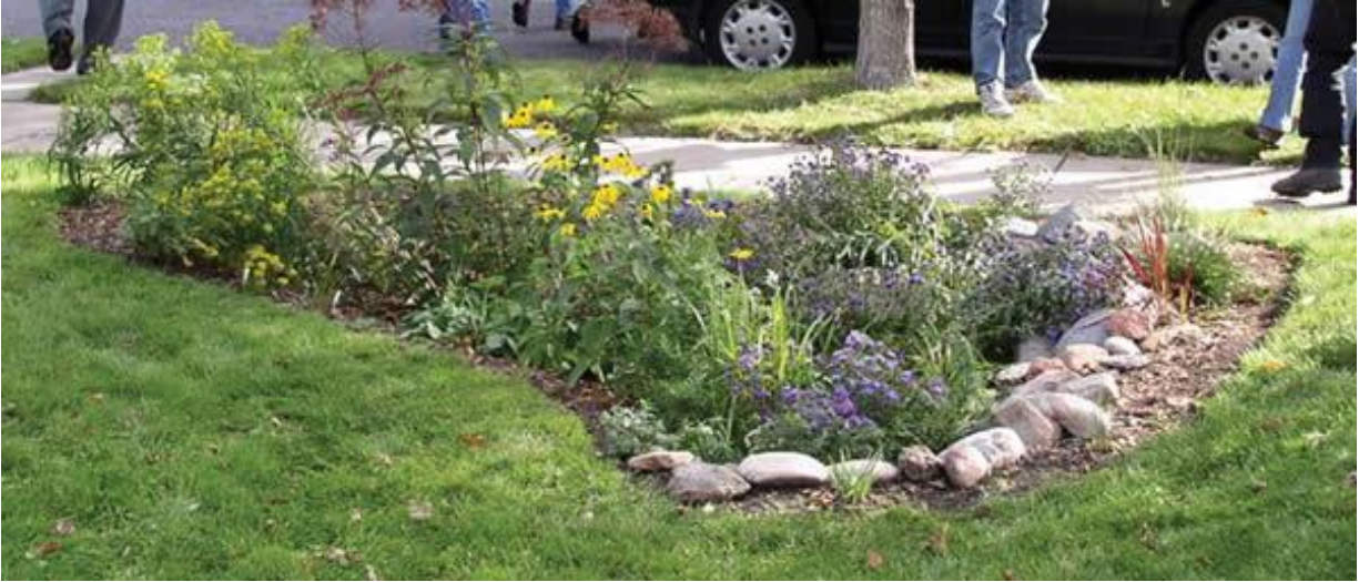
Figure 63: Photo of rain garden
