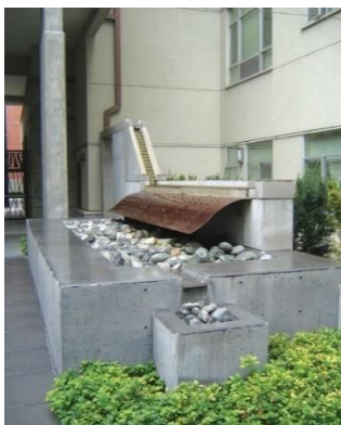
Figure 40: Rain harvesting system on one side of the courtyard (Echols and Pennypacker 2015)
