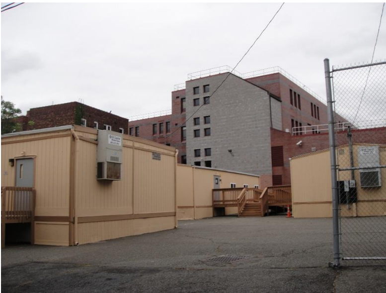
Figure 4-4. Trailer classrooms on the asphalt-paved ground.
