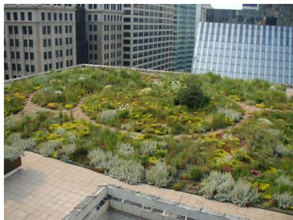
Figure 6.1 Chicago City Hall green roof (Michigan State University, Department of Horticulture, n.d.)
