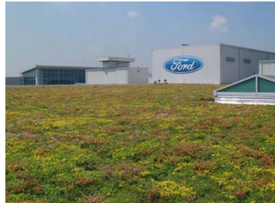
Figure 2.2 Extensive green roof; Assembly Plant, Ford Motor Company, Dearborn, MI (Michigan State University, Department of Horticulture),
