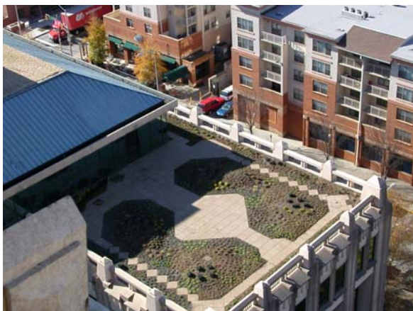
Figure 2.7 Atlanta City Hall green roof; December 2003 (courtesy of Benjamin Taube, Environmental Manager, City of Atlanta).
