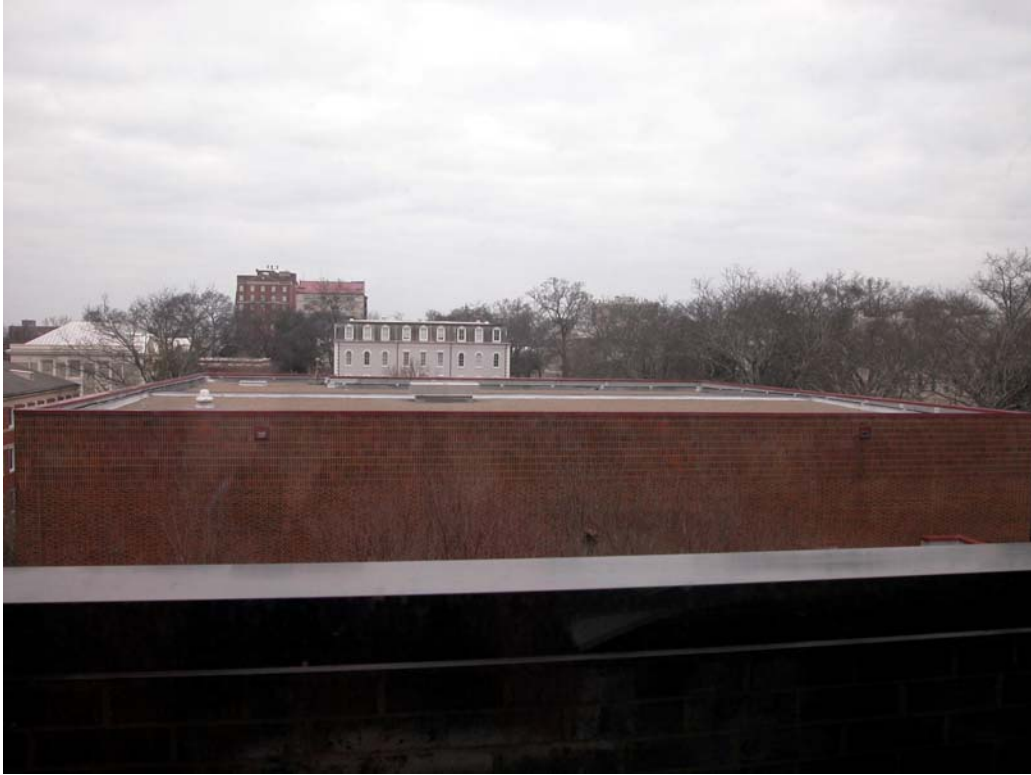
Figure 7.2 View north from the 4 th floor, Caldwell Hall, onto the law school library annex rooftop. Moore College is the white building in the background.
